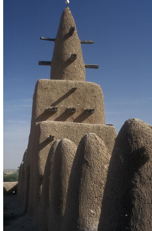
with quantities of chopped straw, dry rice husks, or cow manure, and less commonly with tiny pebbles, ash, earth from termite mounds, powdered baobab fruit, or *kari * (shea-nut) butter. Left to ferment, the additives improve cohesion, durability, and water resistance.
