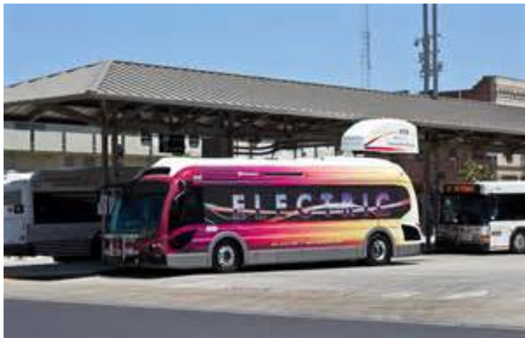
Figure 1. Proterra bus overhead charging station
