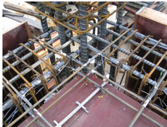
(b) Conflict of EW and NS beams longitudinal bars
