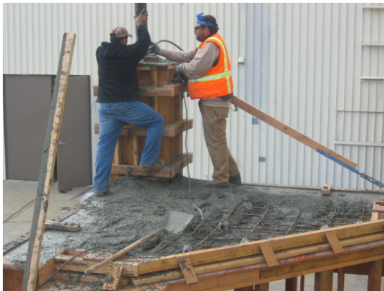
(c) Concrete casting
