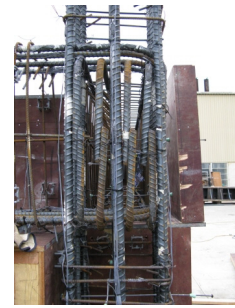
(a) Conflict of the beams and column longitudinal bars
