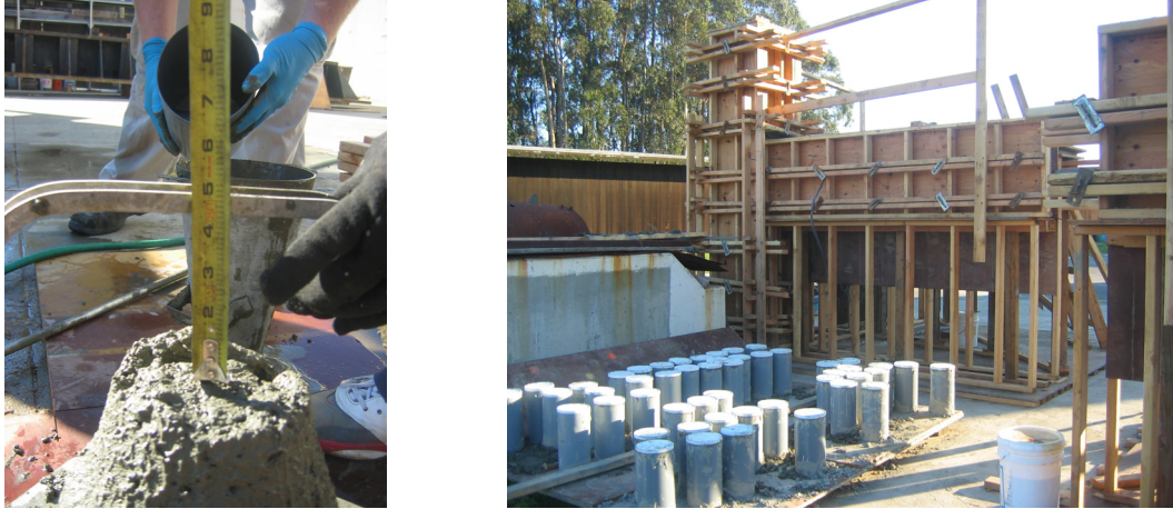
Figure B.1. Slump test and curing.
