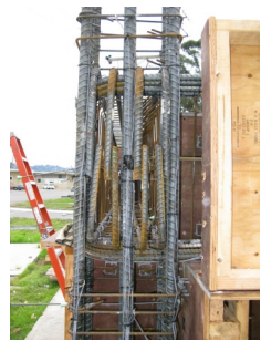
(a) Conflict of the beams and column longitudinal bars
