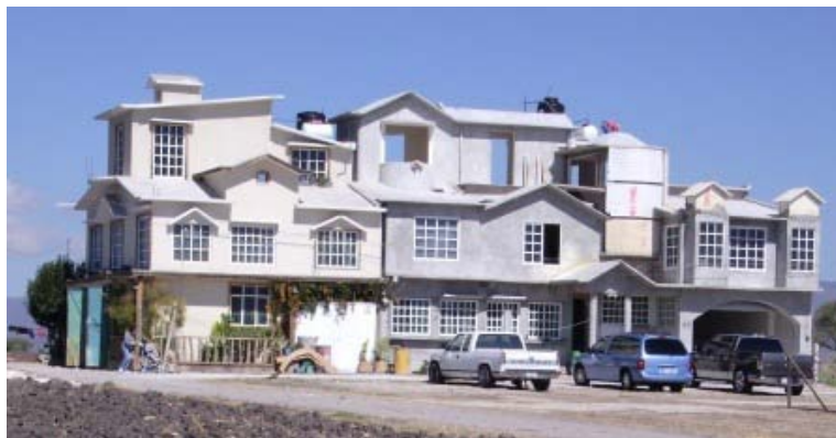
Figure 11. An American-style home under construction in the outskirts of Acámbaro. Photo taken in February 2007 by the author.
