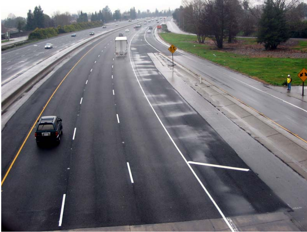
Figure 18. Ponding starting at Station 50+00 (outside lanes, northbound).
