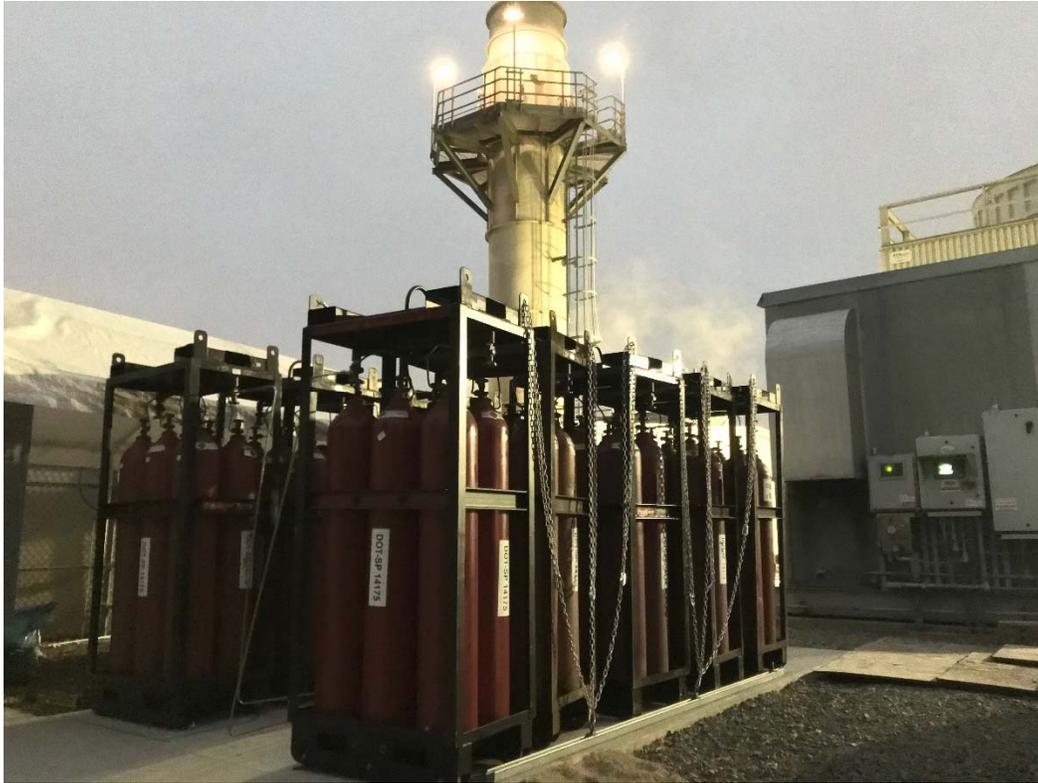
*Figure 88. Siting of the six-pack hydrogen cylinders at the UCI Central Plant on concrete pad space.*
