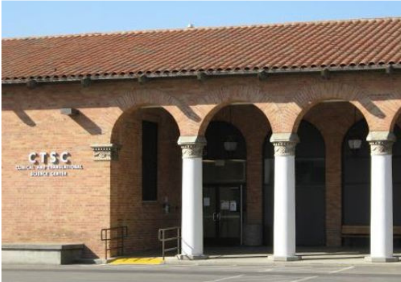
The CTSC facility on the UC Davis Medical Center
