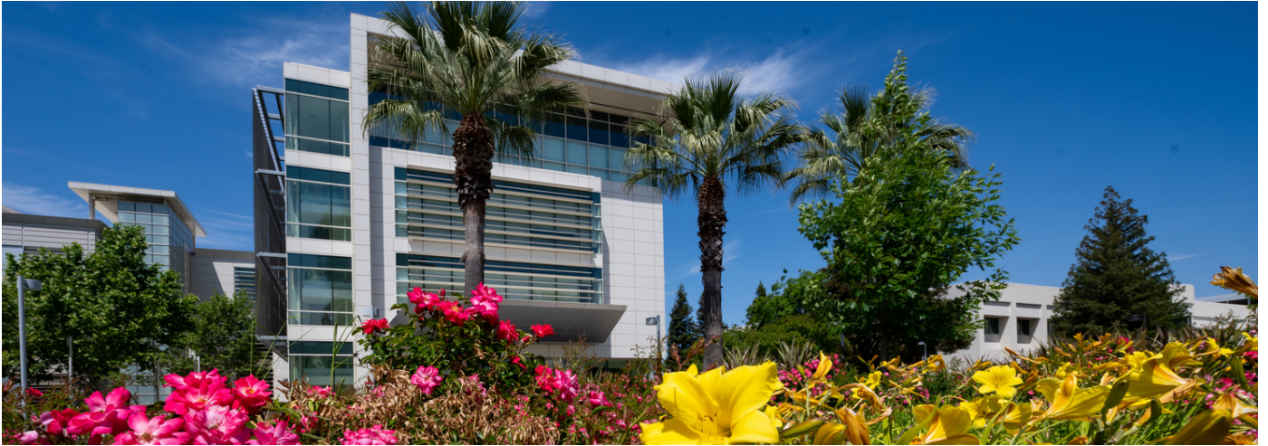
Center for Health and Technology, also housing the Center for Virtual Care
