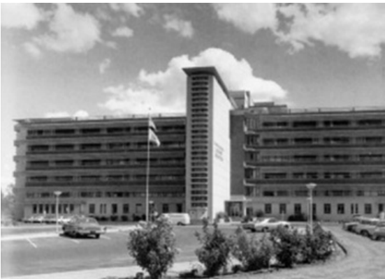
The Sacramento County Hospital in 1972
