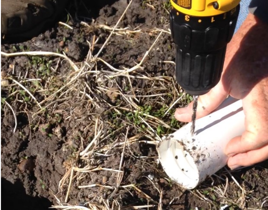
Figure 11 Piezometer preparation. Eight holes were drilled around the base of a two-inch PVC pipe.
