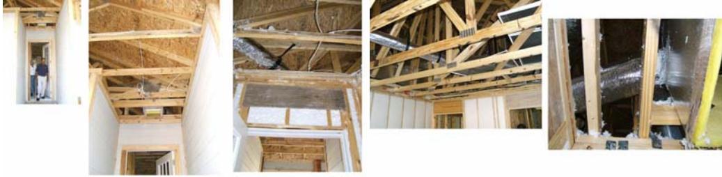
OA Duct connection to Return Air Plenum
