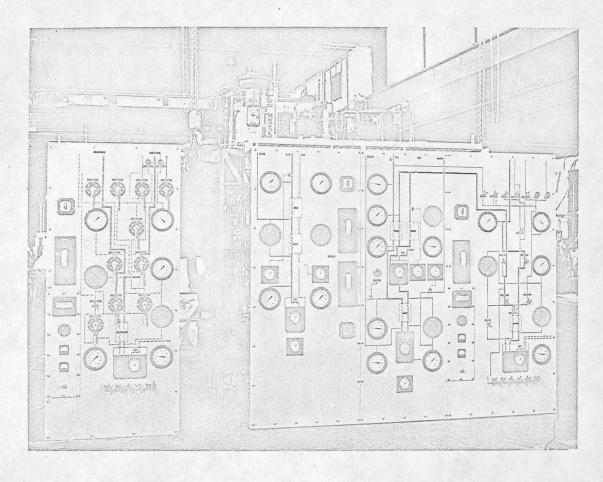
Fig. 34. Hydrogen refrigeration system for the 80-inch Brookhaven bubble chamber. From left to right: low-pressure hydrogen purifier, nitrogen refrigerator-liquefier, hydrogen refrigerator, and high-pressure hydrogen purifier. (Courtesy Cryogenic Engineering Co.)
