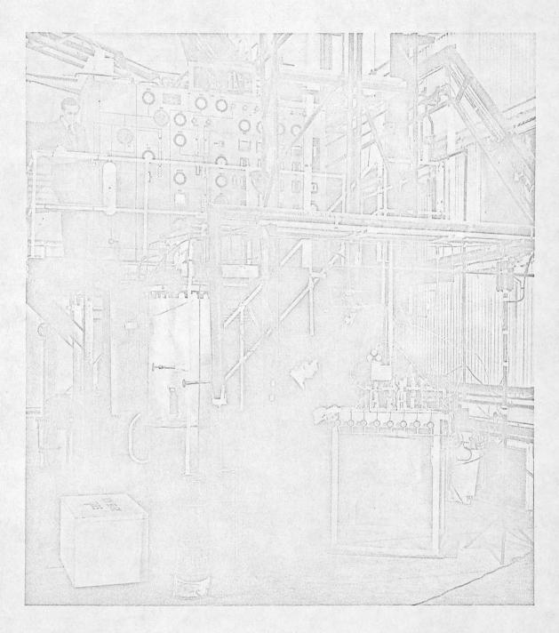
Fig. 33. Refrigerator control board for the 60-inch British National bubble chamber. (Simulated refrigerator load, left foreground; control-valve assembly at right.)
