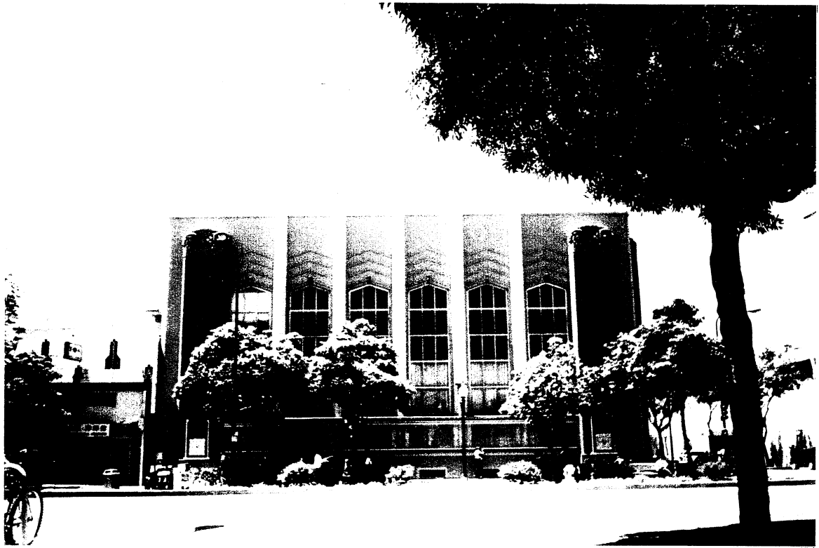
Fig. 2.1 View of Berkeley Public Library from Kittredge St.
