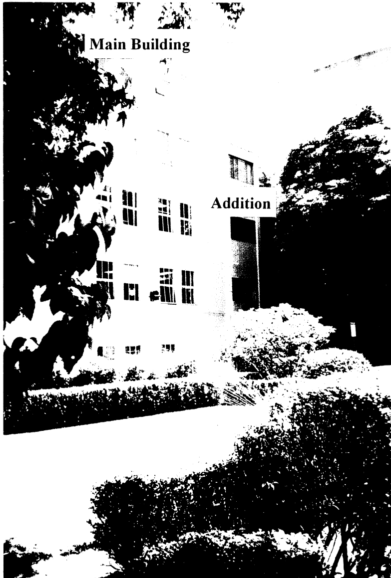
Fig. 2.3 View of Building Addition from the Parking Lot on Kittredge St.
