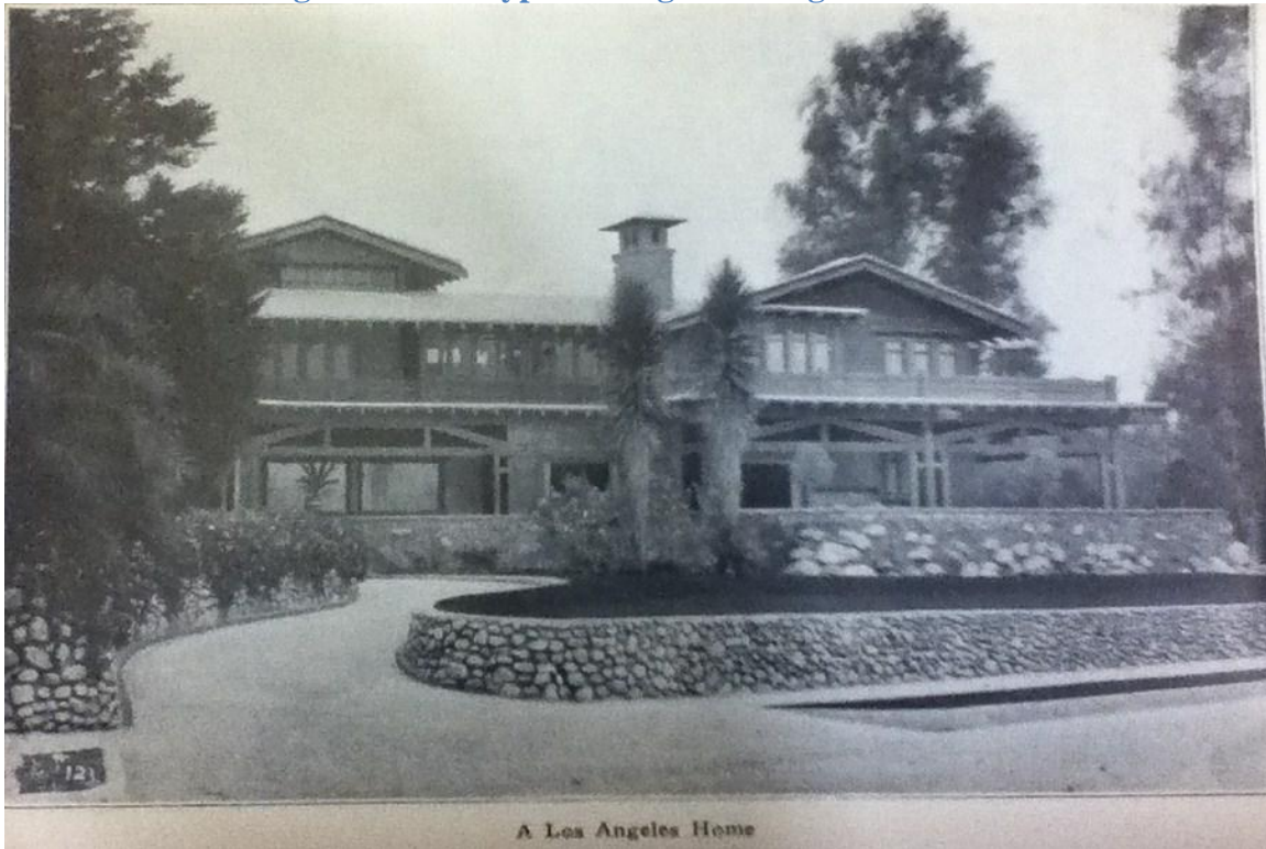
Figure 2.2: A Typical Large Los Angeles Home 10
