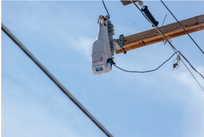
Figure 7-1. “TripSaver” automated recloser
