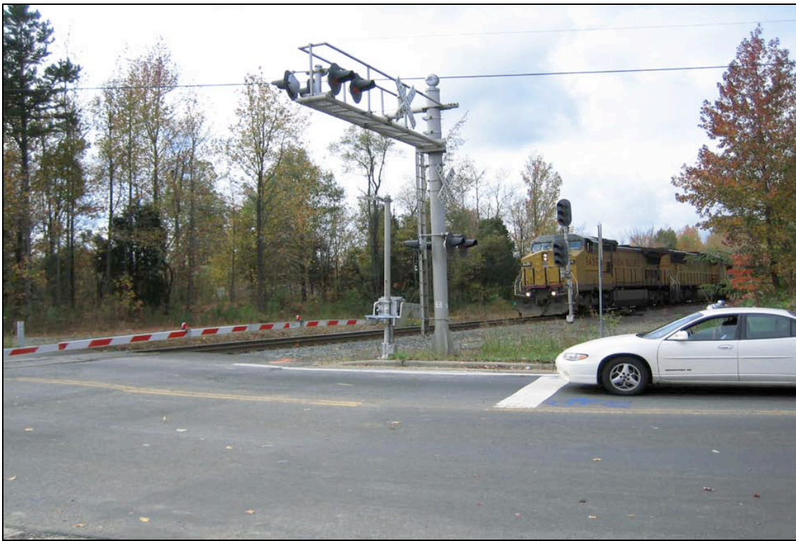
25 FIGURE 7 Longer-Arm Gates at Orr Road, North Carolina 26
