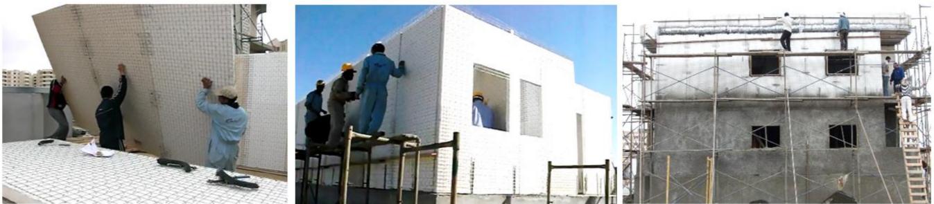
Figure 1. Light-weight feature of CSP building system.
