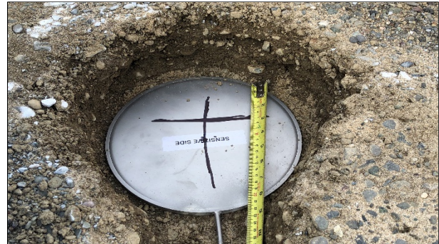
Figure 4.5: Pressure cell installation in the aggregate base.
