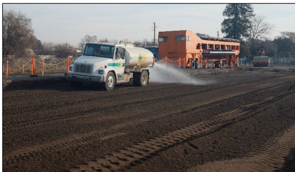
Figure 3.8: Subbase: Water spraying.
