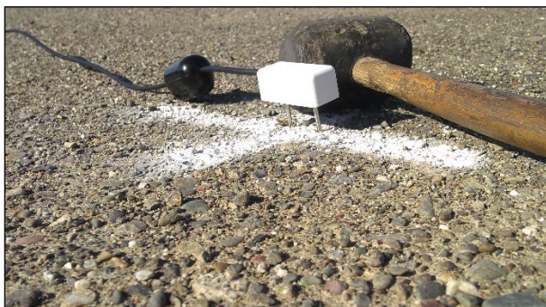
Figure 4.6: Moisture sensor installation on top of subbase.
