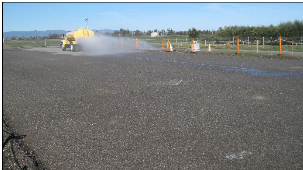
Figure 3.16: Base: Water spray prior to prime coat application.
