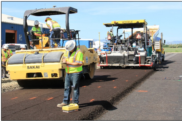
Figure 3.25: CCPR: Paving and breakdown compaction.
