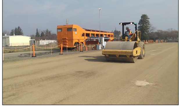
Figure 3.14: Base: Final compaction.
