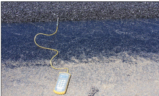
Figure 3.38: RHMA-G: Temperature measurement with thermocouple.
