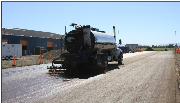
Figure 3.29: CCPR: Curing seal application.
