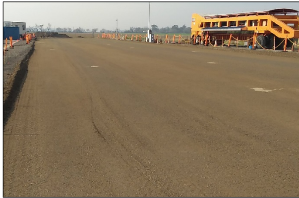
Figure 3.15: Base: Completed preparation.
