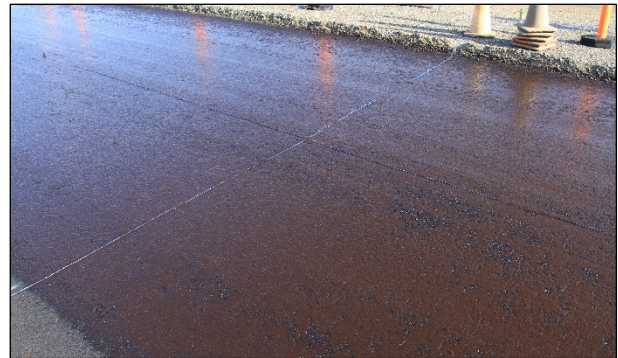
Figure 3.32: RHMA-G: Close-up view of tack coat application.
