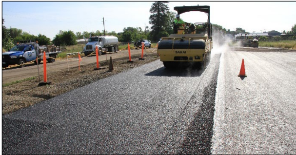
Figure 3.35: RHMA-G: Breakdown compaction.
