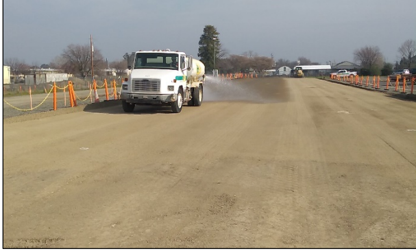
Figure 3.13: Base: Water spraying.
