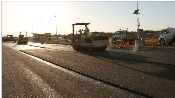
Figure 3.37: RHMA-G: Final compaction.
