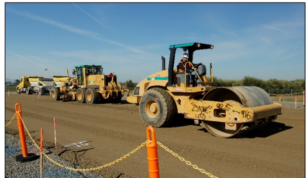
Figure 3.12: Base: Spreading and compacting.
