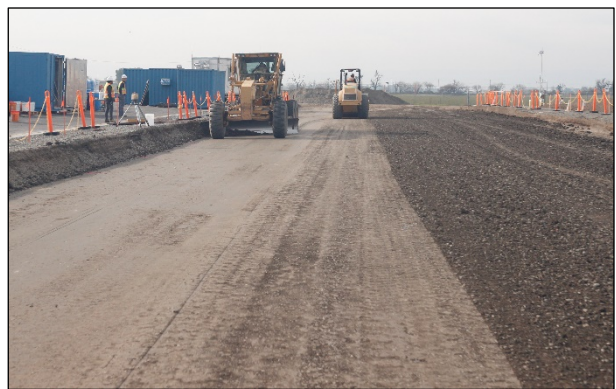
Figure 3.4: Subgrade: Final shaping and compaction.
