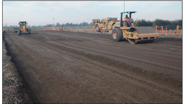
Figure 3.7: Subbase: Spreading and compacting.
