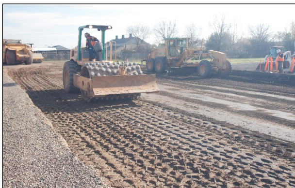
Figure 3.3: Subgrade: Padfoot roller compaction.
