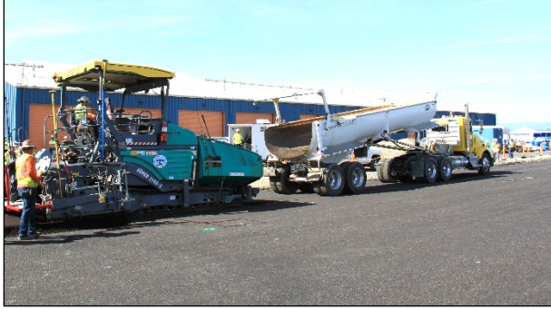
Figure 3.23: CCPR: Material delivery with long-bed dump truck.
