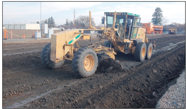
Figure 3.2: Subgrade: Mixing and shaping.
