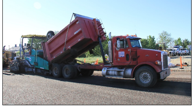
Figure 3.24: CCPR: Material delivery with short-bed dump truck.
