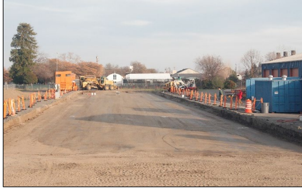
Figure 3.5: Subgrade: Completed preparation.
