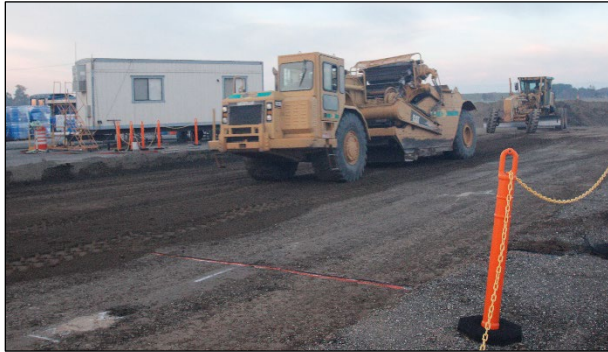
Figure 3.6: Subbase: Importing and spreading material with a scraper.
