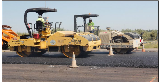
Figure 3.36: RHMA-G: Intermediate (front) and final compaction (back).
