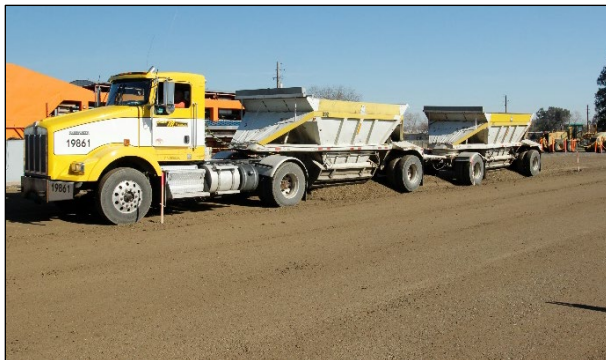
Figure 3.11: Base: Dumping imported material.
