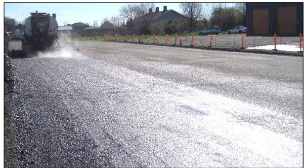
Figure 3.17: Base: Prime coat application.
