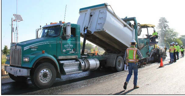
Figure 3.33: RHMA-G: Dumping mix into the paver.
