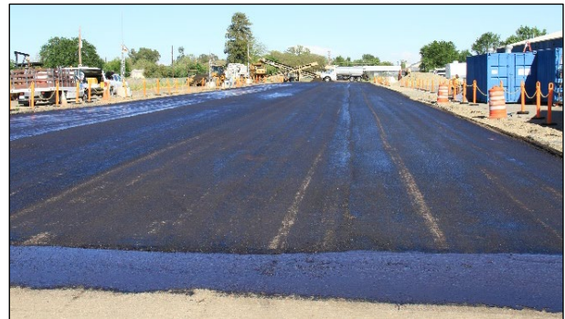
Figure 3.30: CCPR: Completed recycled layer after construction.
