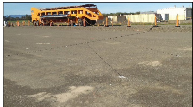
Figure 4.7: Moisture sensor locations on top of subbase.
