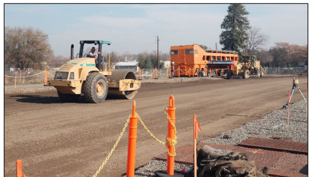
Figure 3.9: Subbase: Final shaping and compaction.
