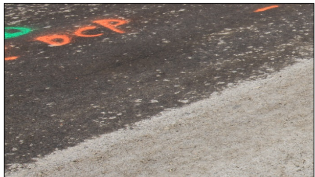
Figure 3.28: CCPR: Crack-free surface after final compaction.
