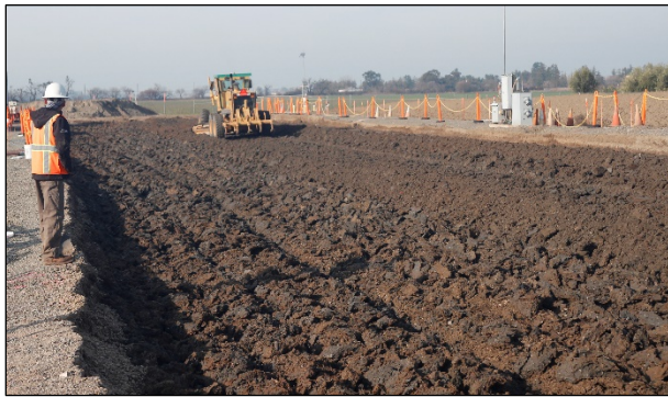
Figure 3.1: Subgrade: Ripping with a grader.
