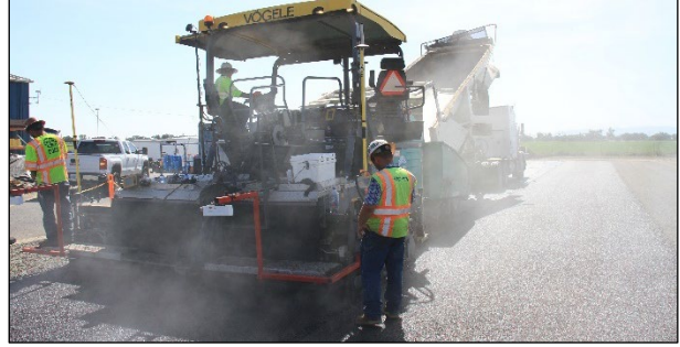
Figure 3.34: RHMA-G: Paving RHMA-G.
