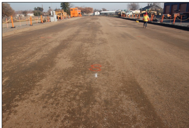
Figure 3.10: Subbase: Completed preparation.
