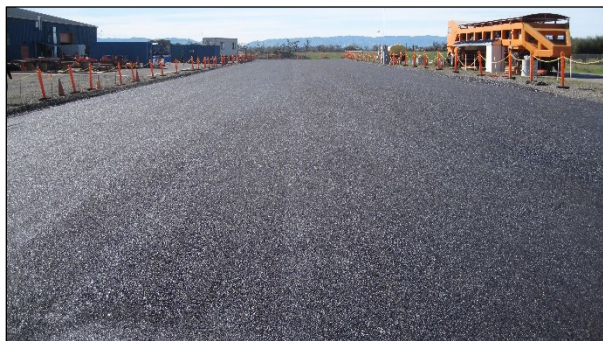
Figure 3.18: Base: Completed prime coat application.
