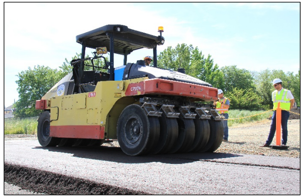
Figure 3.26: CCPR: Intermediate compaction with pneumatic tired roller.
