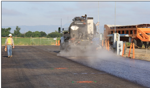
Figure 3.31: RHMA-G: Tack coat application.
