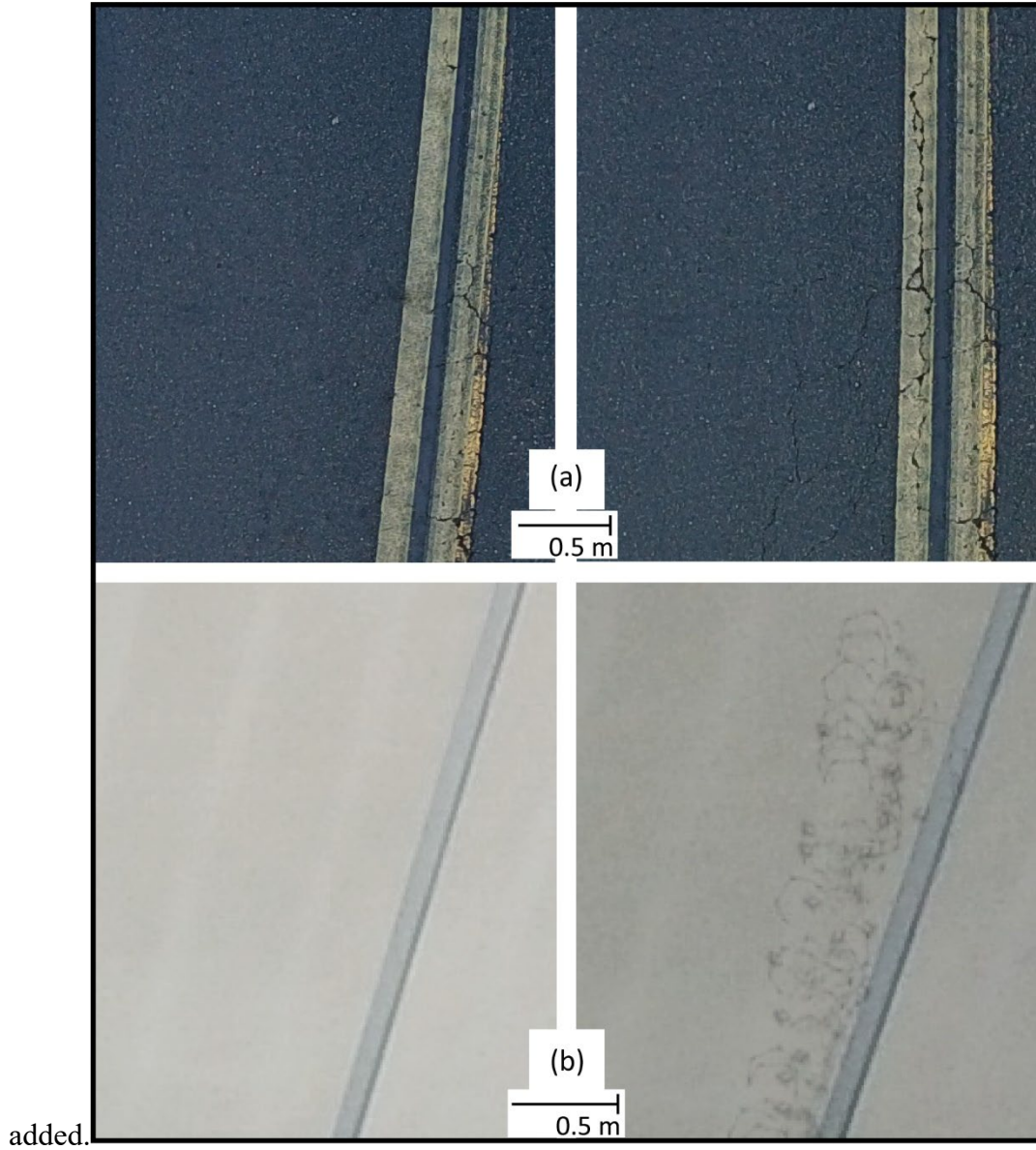
Figure II.1. Examples of damage simulation in baseline (left images, (a) and (b)) and time- n (right images, (a) and (b)) pairs. Removal of cracks in baseline images is shown (top) and addition of cracks to time- n images is shown (bottom).
