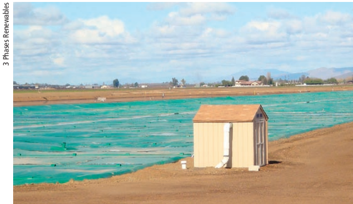
Hilarides Dairy in Lindsay, Calif., has installed covers on its manure lagoons to capture methane for electricity generation and vehicle fuel. The dairy hopes to capture the economic value of destroying methane by selling carbon offsets once the market is established.
