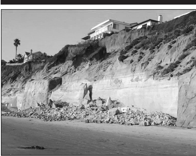
Figure 1. Seacliff failure in Solana Beach, September 28, 2004.
