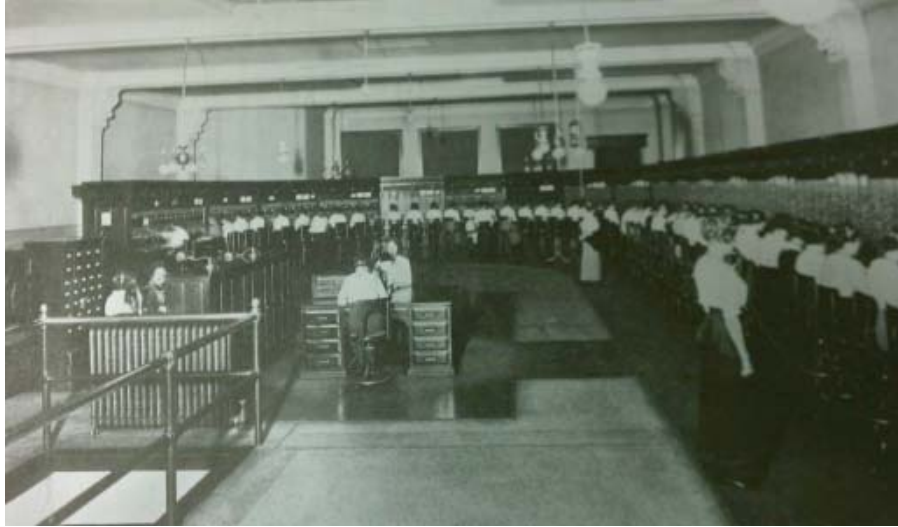
A U-shaped Bell System operating room, 1914. This design commonly existed since at least 1906. A Bell employee describes this as “a typical exchange.” The chief operator, sitting in the middle, oversees the standing assistant supervisors who oversee the operators facing the walls. 498
