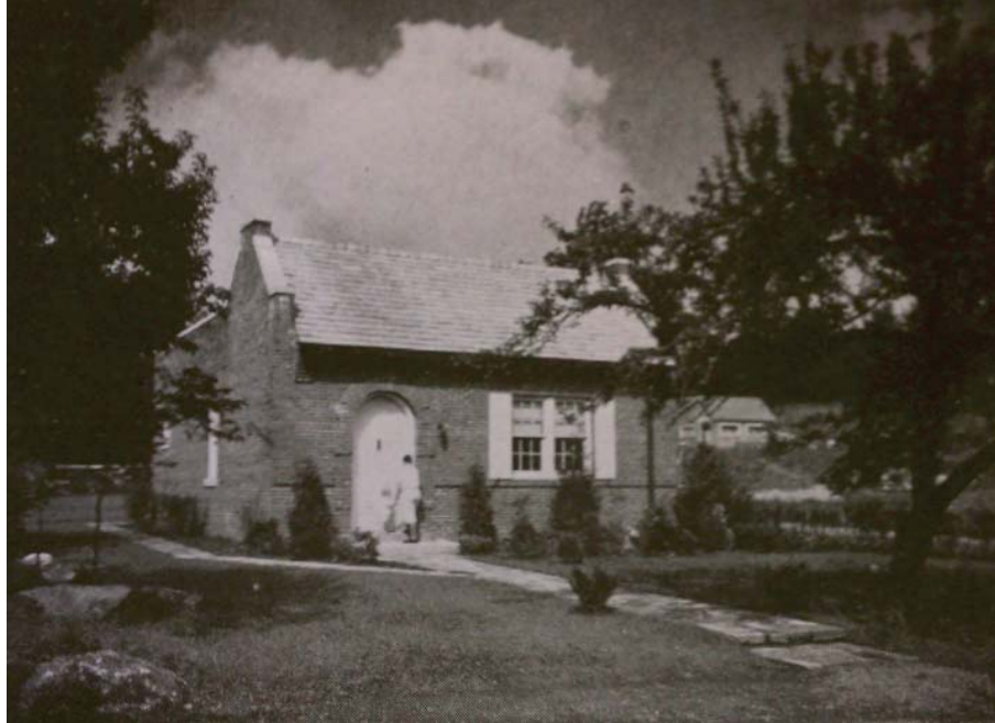
A telephone switching station in Armonk, New York, 1931. Despite the fact that a mother and child are seen approaching this building, no one worked here. Nonetheless, the building still featured a stone path, an arched door, windows with shutters, and attentive landscaping. 1931. 579
