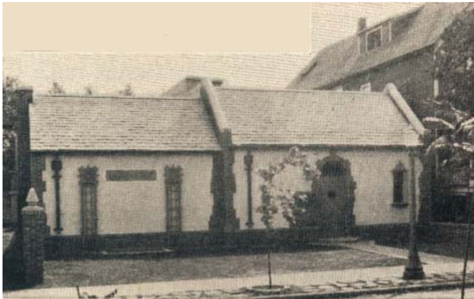
An unoccupied electrical substation built by the Commonwealth Edison Company in the residential neighborhood of Windsor Park, Chicago, 1929. 578
