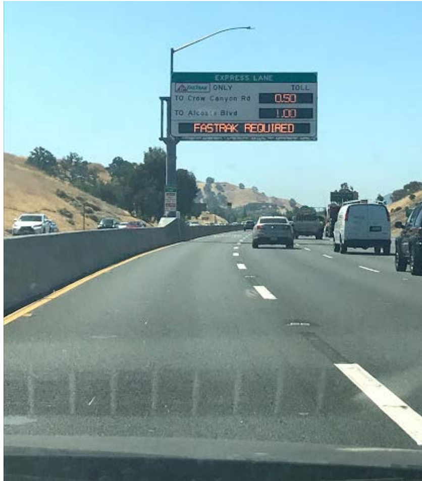
Fig 4. Left Shoulder of the I-680 Express Lane.
