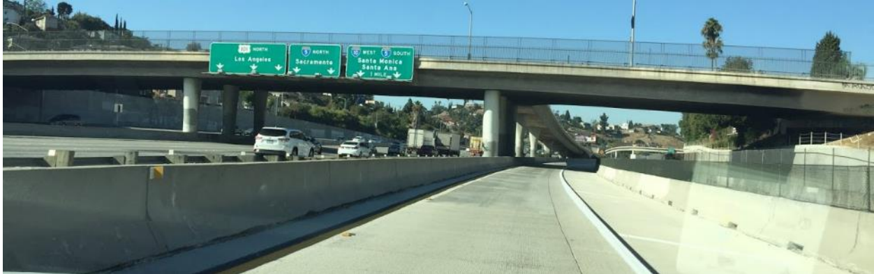
Fig 10. Beginning of the I-10 Express Lane.
