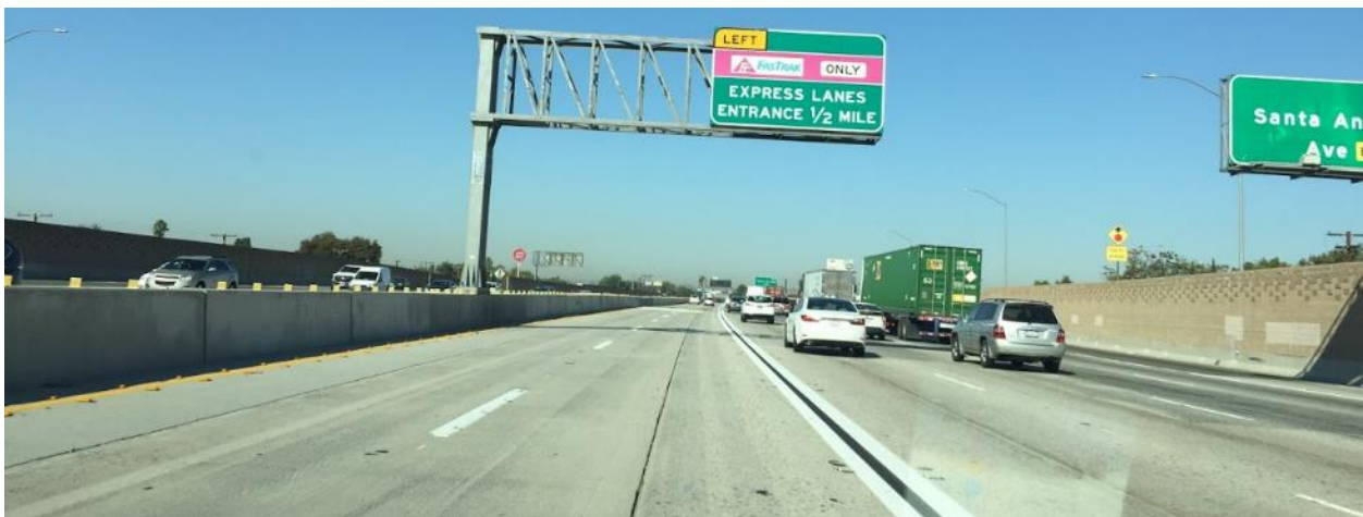
Fig 11. Two-Lane Segment of the I-10 Express Lane Facility.
