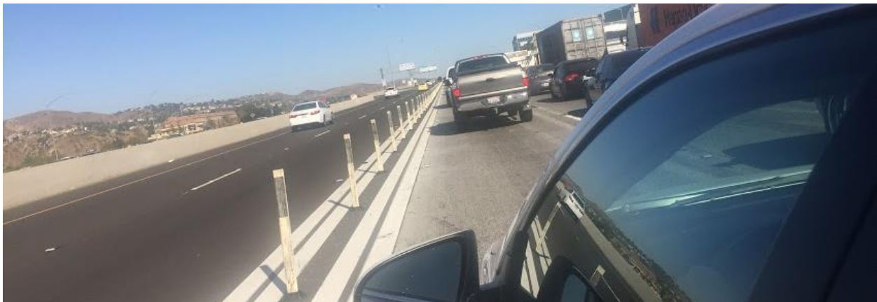
Fig 16. Removable Segregation for SR-91 Express Lane.
