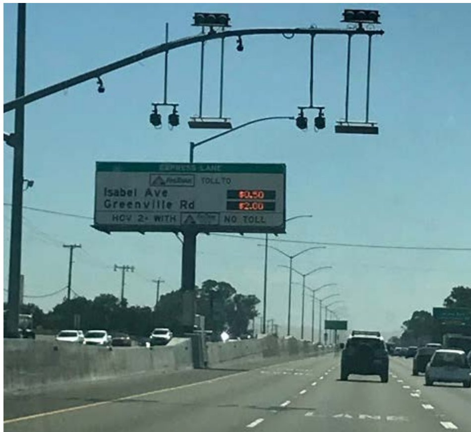
Fig 6. The two-lane facility of the I-580 Express Lane.
