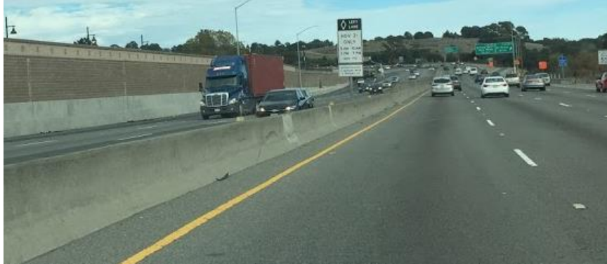
Fig 2. Left Shoulder of the I-80 HOV Lane.
