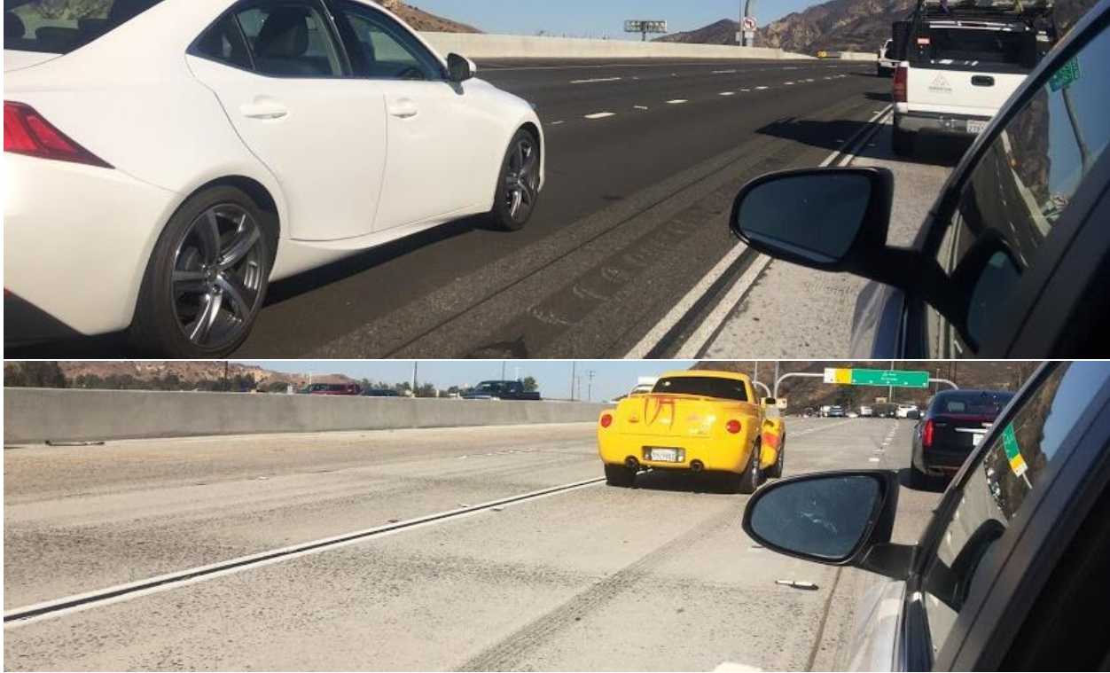
Fig 17. Ingress/Egress Section of SR-91 Express Lane Facility.
