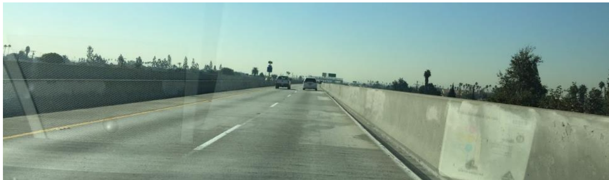
Fig 14. Elevated Express Lane Facility on I-110.
