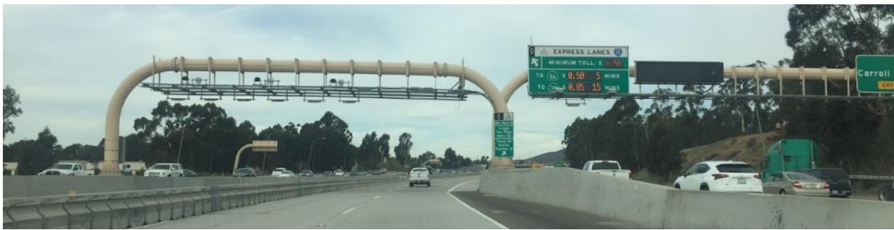
Fig 23. Changeable Message Signs on I-15 Express Lane.
