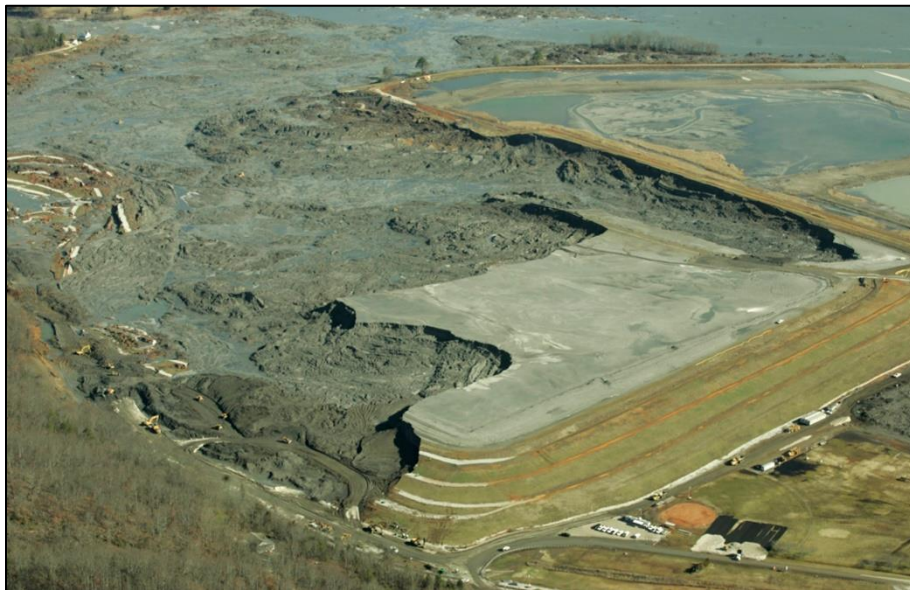
Figure 1. Failed fly ash impoundment at Kingston Fossil Plant, TN (Photo: Greenpeace).
