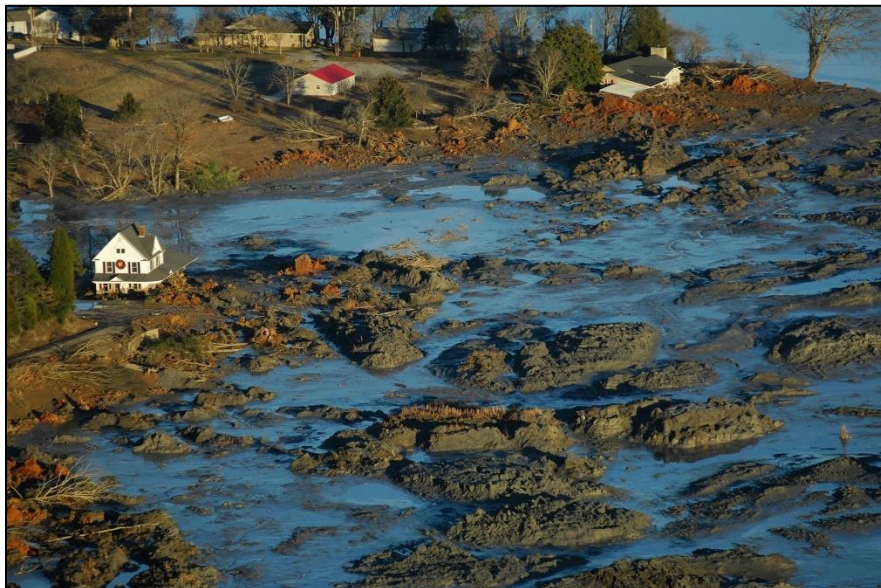
Figure 2. Fly ash material that flowed downstream of the failed impoundment (Photo: National Geographic).
