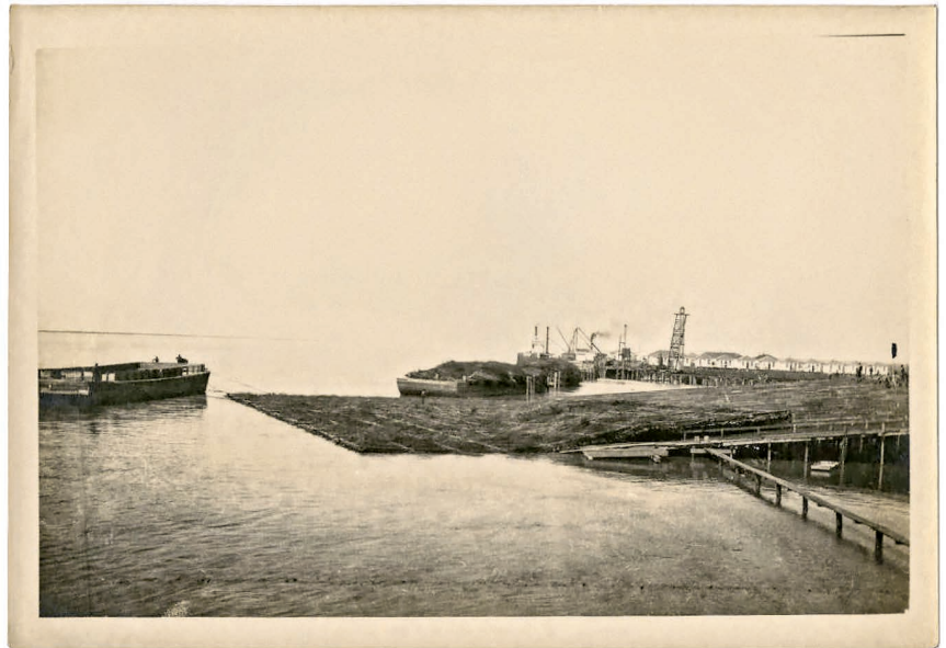
Figure 9 Burrwood, Louisiana, and Southwest Pass jetties construction photographs, circa 1905–1915. The photograph shows the construction process at the Southwest Pass using the mattress systems prototyped at the South Pass more than 30 years earlier by Eads. The wood and brush mattress was assembled on a platform and floated into position with tugboats. (Source: Burrwood, Louisiana, and Southwest Pass Jetties Construction Photographs, Mss. 5068, Louisiana and Lower Mississippi Valley Collections, LSU Libraries, Baton Rouge, Louisiana, USA)
