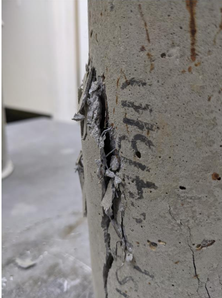
Figure 4-11. The fracture surface for a fiber-reinforced concrete after compression test.
