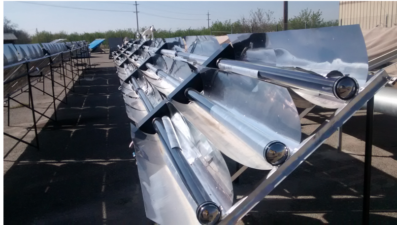
FIGURE 1.2: Solar thermal Compound Parabolic Concentrator
