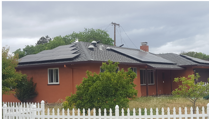
FIGURE 1.1: Flat rooftop PV solar panels
