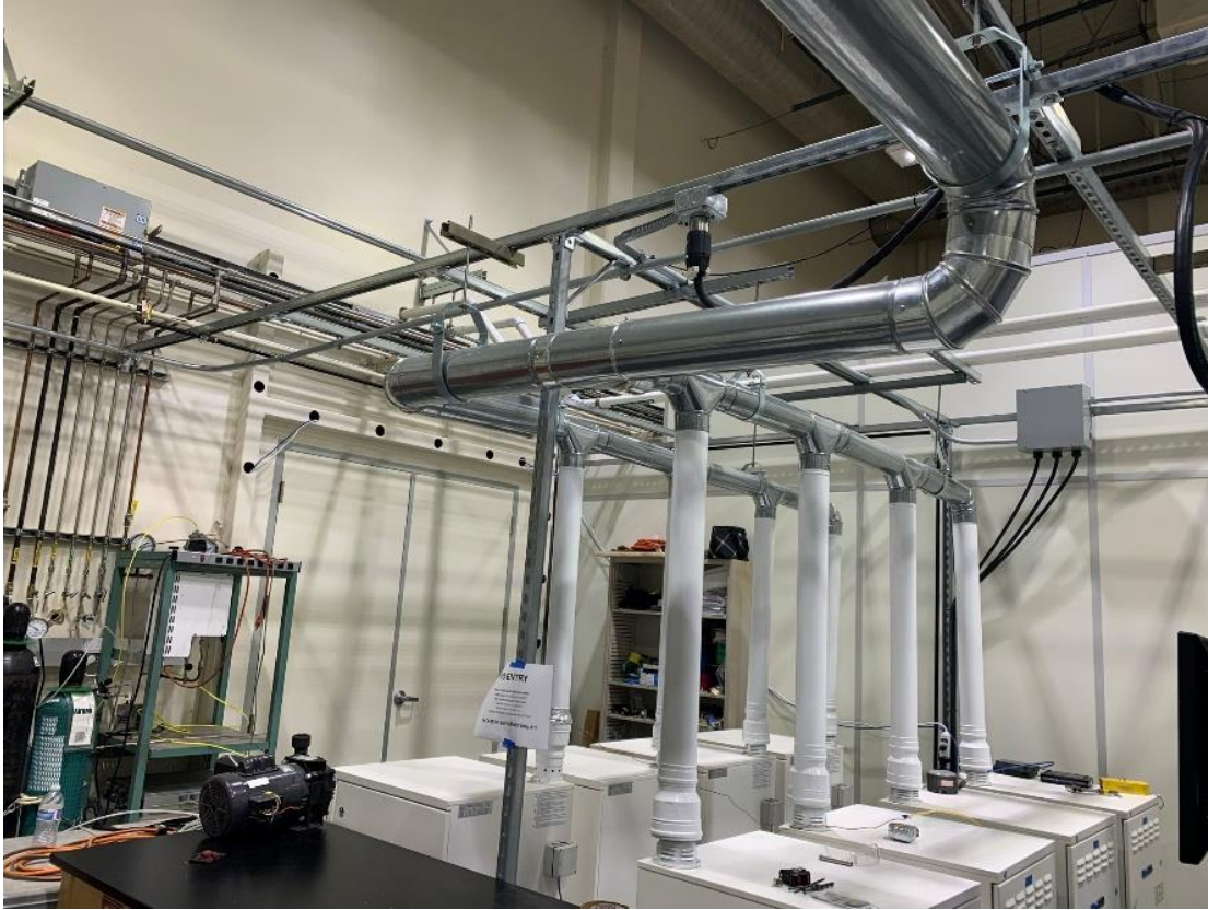
Figure 91. BlueGEN exhaust manifold.
