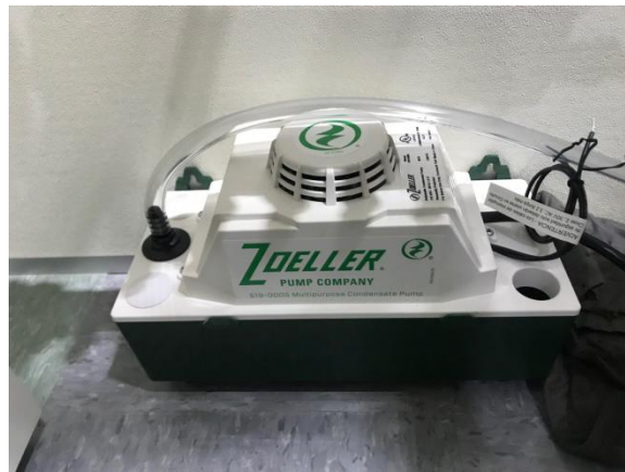
Figure 89. Pump used for fuel cell water rejection connection.
