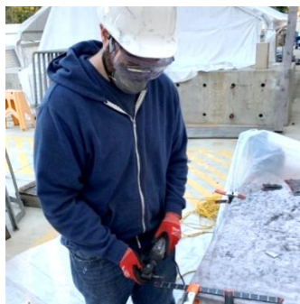
Figure 6-3: Cutting of CFRP Composite Laminate
