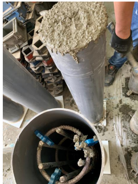
b) Casting of RC Columns
