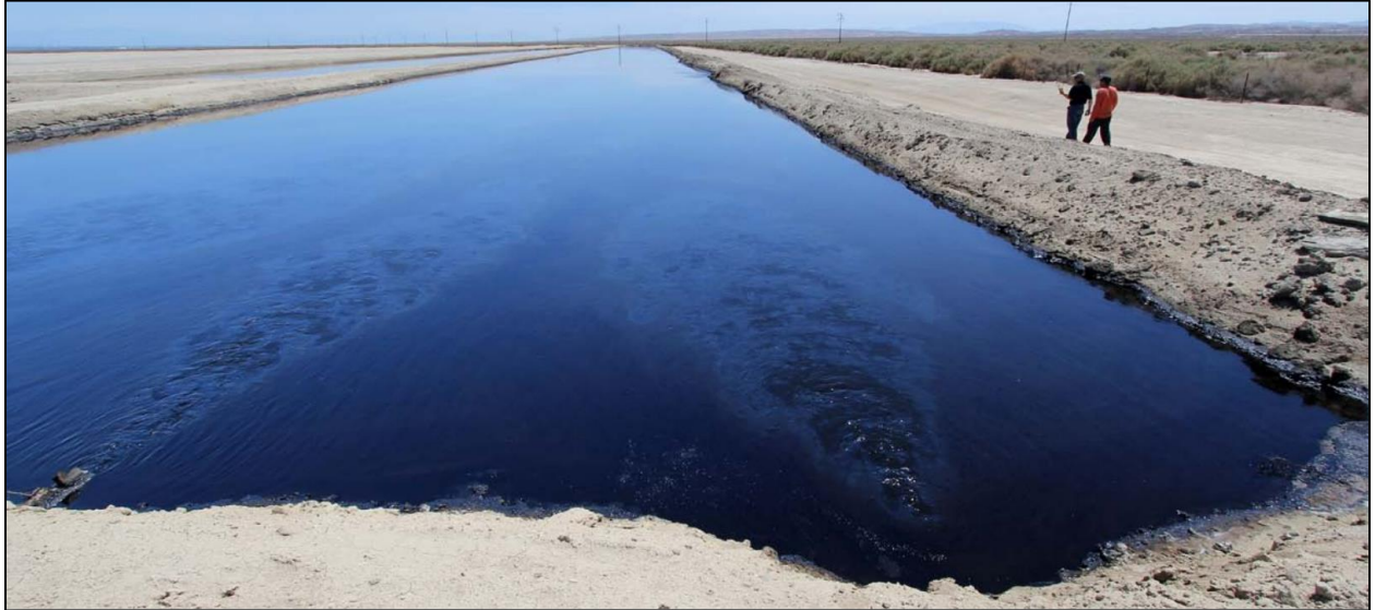
Figure 108: Unlined Wastewater Storage Pit 1 in Kern County, California.
