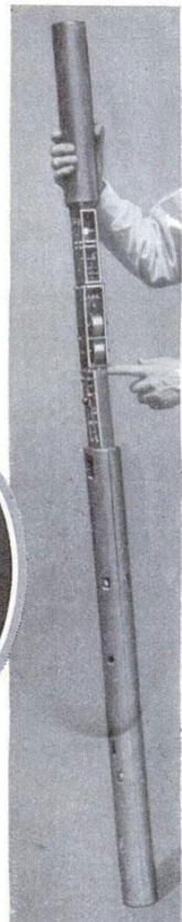
In circle, camera that makes records of film showing the inclination of well being dug. Right, whipstock that is set at bottom of well to deflect bit. Left, acid-etched bottle that shows slant of the well
