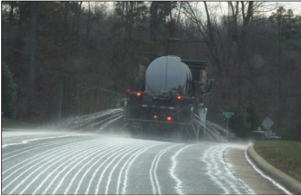
Figure 26: Spraying Wastewater Brine as a De-Icing Treatment in West Virginia.
