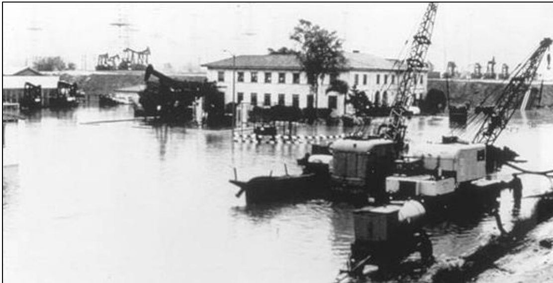
Figure 77: Tidal Flooding from Land Subsidence at the Wilmington Oil Field, Circa 1950s.
