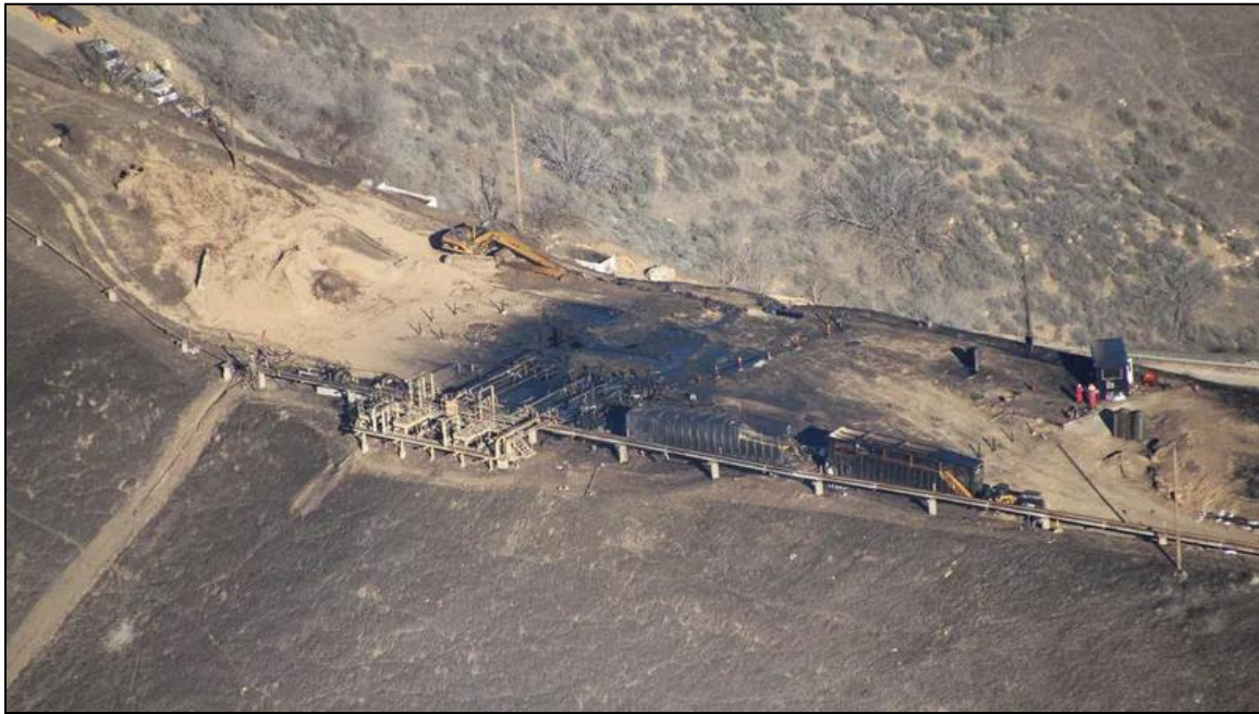
Figure 144: Aliso Canyon Storage Facility Blow Out Site, December 2015.
