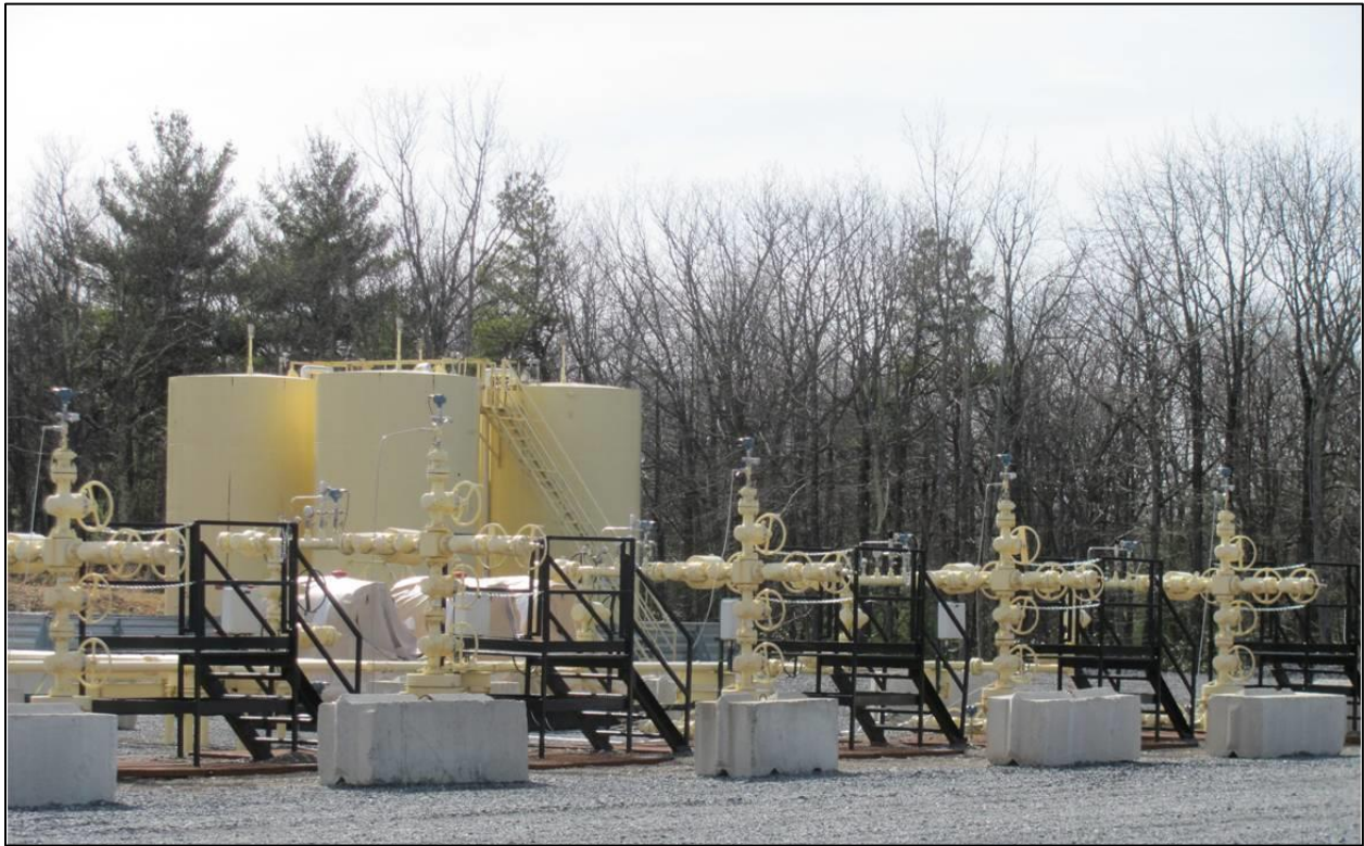
(Image Source: Anadarko Petroleum Corp., 2014).
