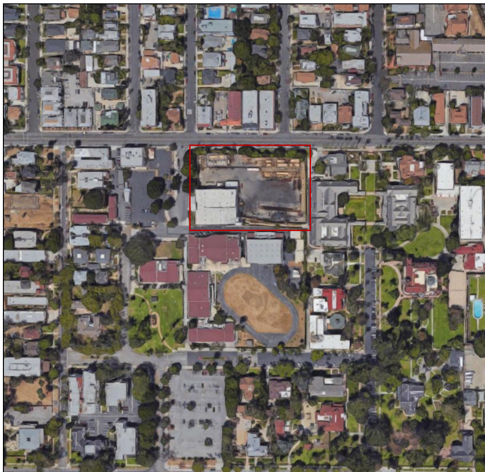
Figure 100: AllenCo Energy Site in University Park Neighborhood, Los Angeles.
