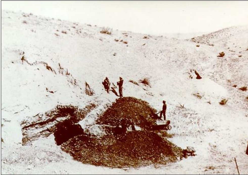
Figure 36: Asphaltum Excavation in McKittrick, California.
