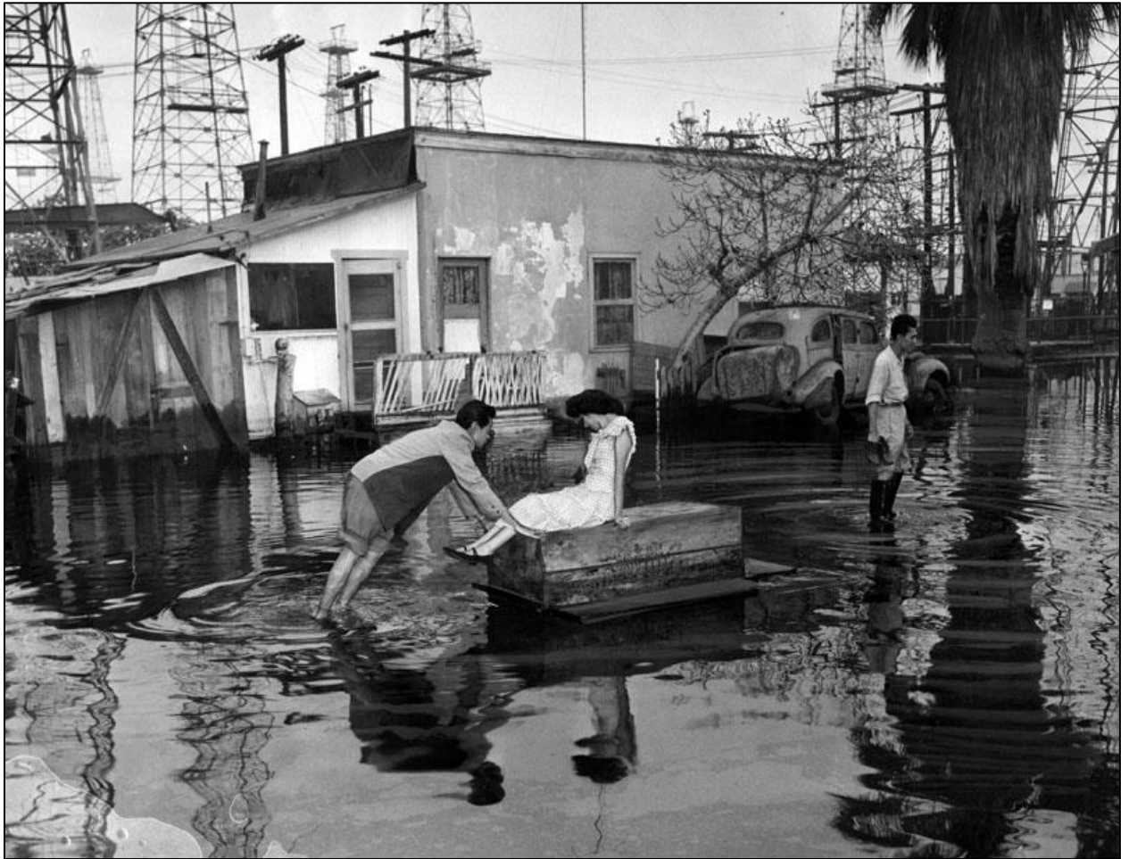
Figure 15: Long Beach Harbor Region High Tide Flooding from Land Subsidence, 1953.
