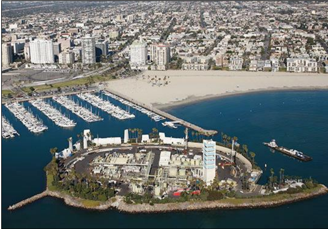
Figure 70: THUMS Offshore Facility Grissom Island at Long Beach Harbor.
