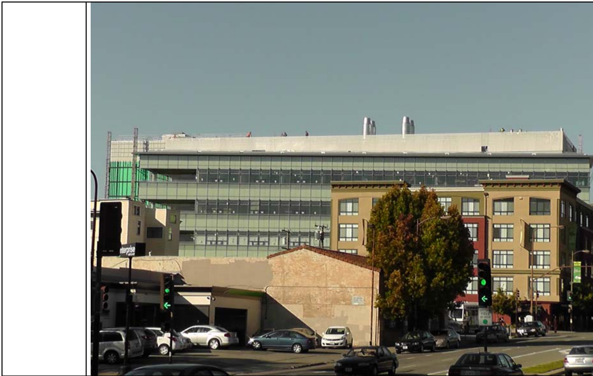
Picture 5 (top) South facade of the Helios building with location of several offices. Caused by the construction process still without sunshades, but already with a clear division between transparent and opaque glazing areas for every floor.
