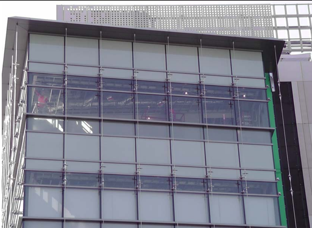
Picture 4 The façade consist of a change between transparent and opaque glazing areas.
