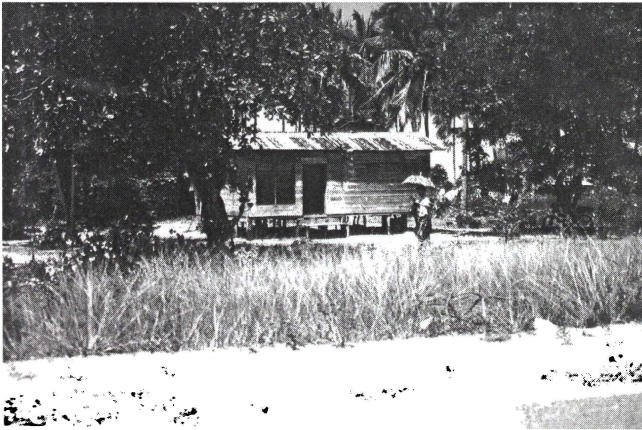
Figure 6: Attap House from Bintan Island near Singapore and Similar to Pre-Independence Singaporean Houses
