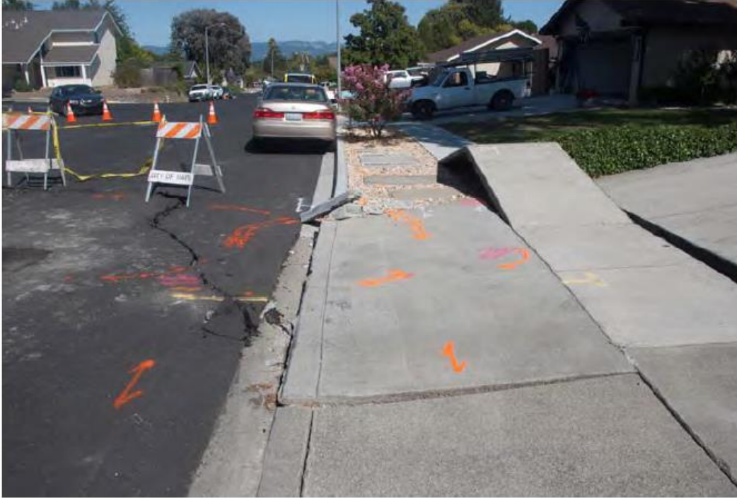
Fig. 2.3. Example of a sidewalk buckling in response to compressional ground movement during the 2014 South Napa, California, earthquake. Image courtesy of NSF-Sponsored GEER Report #GEER-037 (Bray et al. 2014).
