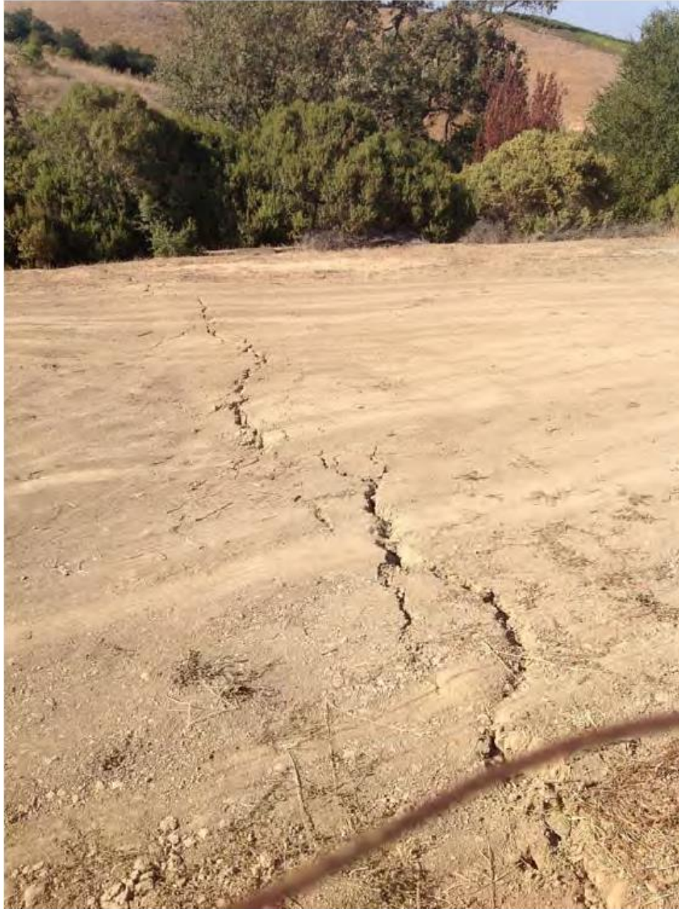
Fig. 2.1. Surface fault rupture trace showing left-stepping en echelon fractures from the 2014 South Napa, California, earthquake. Image courtesy of NSF-Sponsored GEER Report #GEER-037 (Bray et al. 2014).
