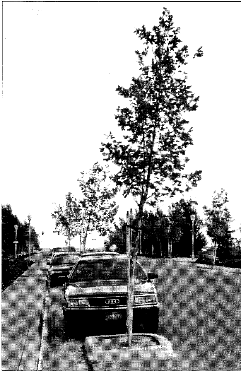
Figure 25: In Laguna West street trees on major streets are placed in wells that project into the street space to break up the parking strip. When the trees mature they will create the sense of a narrower street.
