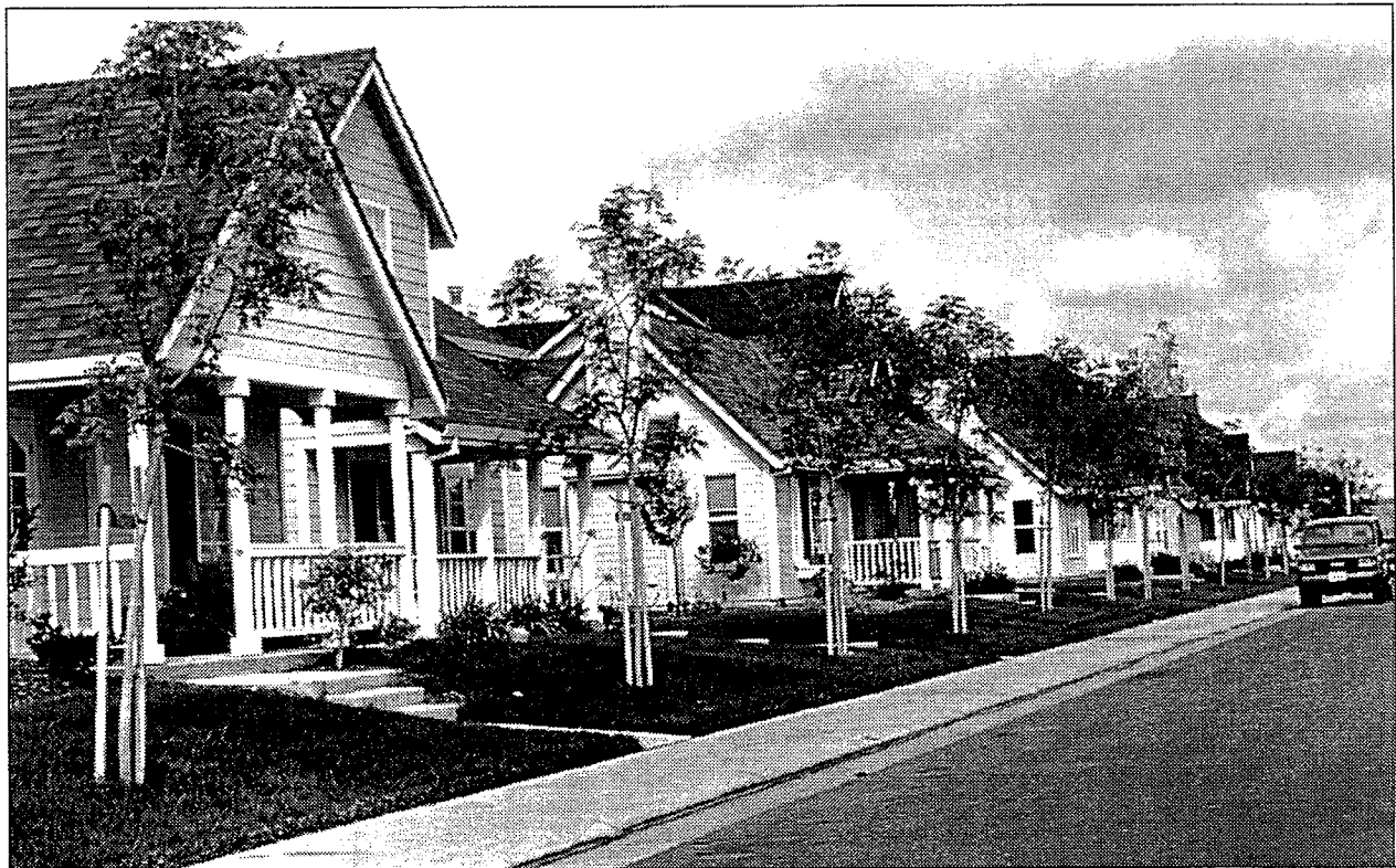
Figure 12: Most homes in Laguna West have front porches, and garages are set to the side or back to avoid the “garagescape” street image.
