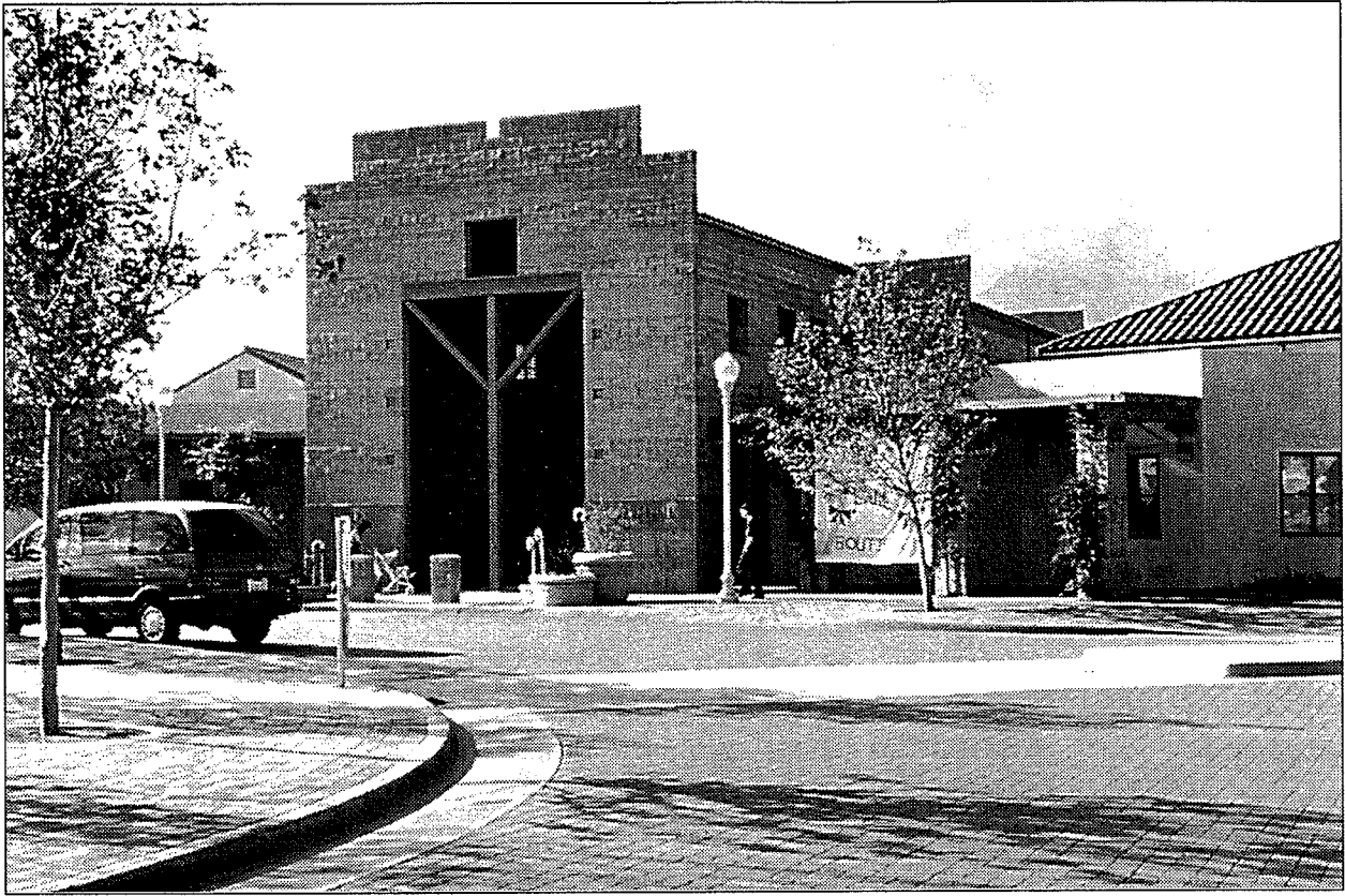
Figure 7: Community Center, Laguna West
