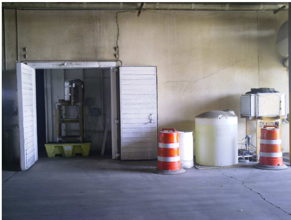
Figure 4.11: Final setup of the system
