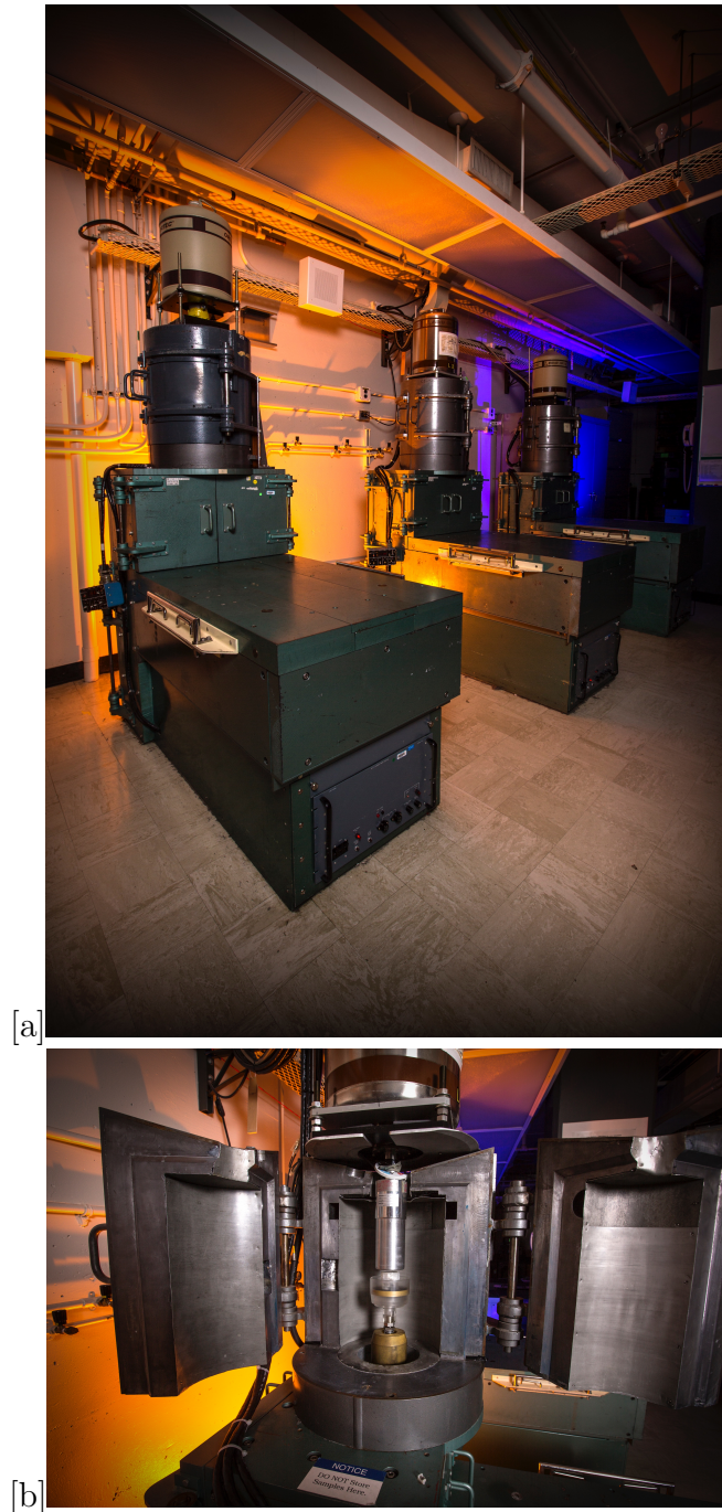
Figure 6.2: a) HPGe room at LLNL, b) HPGe detector.
