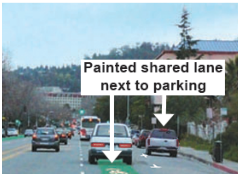
Figure 30. Green painted shared lane marking next to on-street parking
