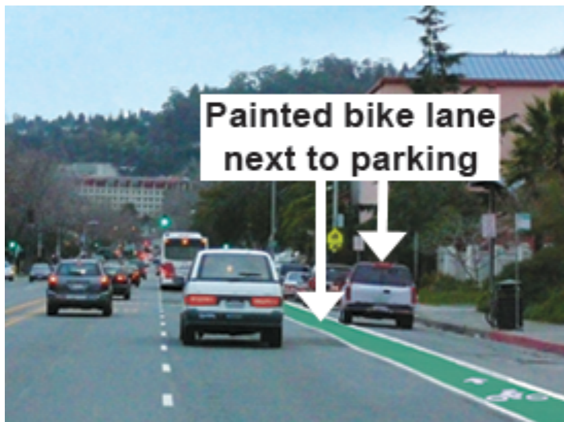
Figure 27. Green painted bicycle lane next to on-street parking
