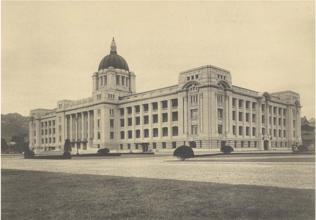
Figure 17. Georg De Lalande and Nomura Ichiro, Japanese General Government Building, 1916-1926 (demolished 1995-1996), Seoul, South Korea.
