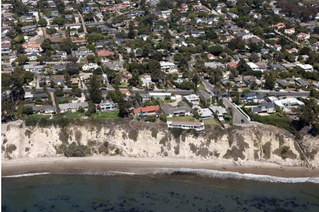
Figure 2.8: Structures along the Mesa That Are Virtually at the Cliff's Edge
