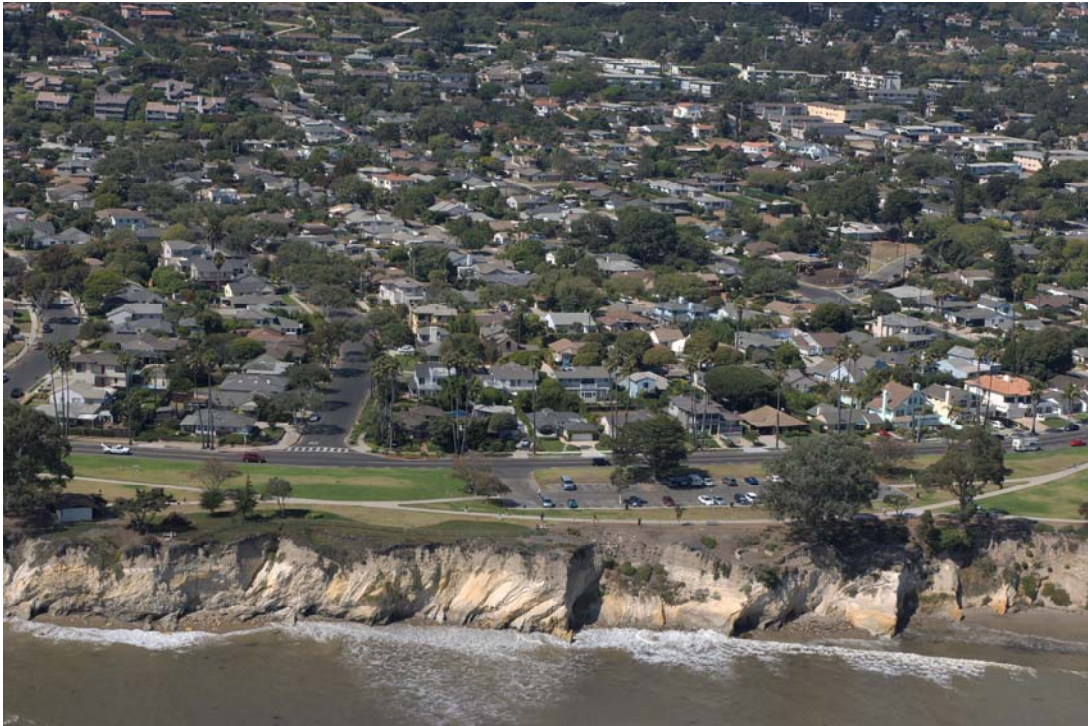
Figure 2.6: Dip Slope in the Monterey Shale along the Shoreline Park Coastline, which Produces Conditions That Are Conducive to Slope Failure
