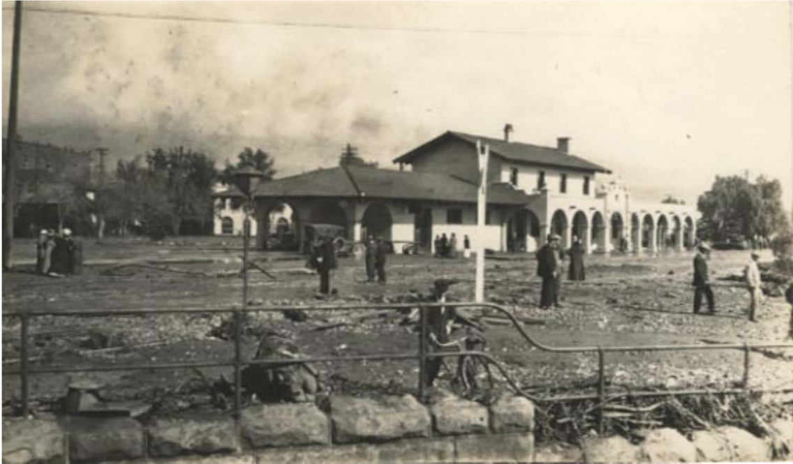
Figure 2.18: Southern Pacific Railroad Station Inundated with Mud Following Flooding in 1914
