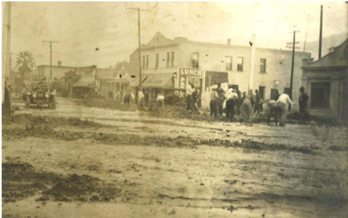
Figure 2.19: Mud Deposited at State and Yanonali Streets during Floods of 1914
