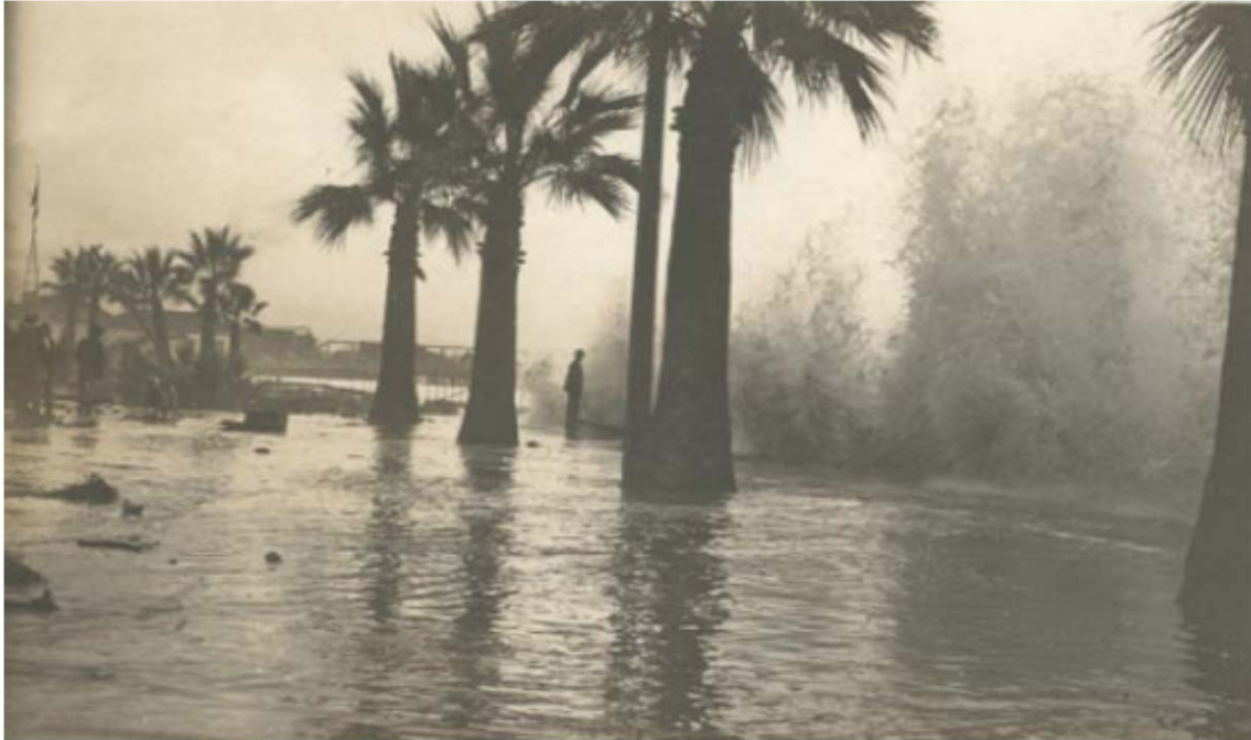
Figure 2.13: Waves Overtopping West Cabrillo Boulevard in 1914
