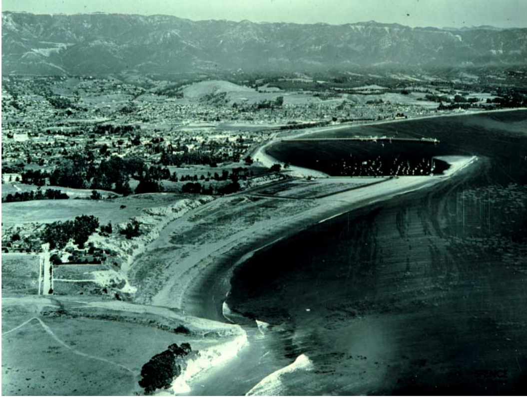
Figure 4.2: Santa Barbara Breakwater in 1930. The connection of the breakwater to Cabrillo Point serves as a dam and allows the area upcoast of it (to Ledbetter Point) to trap a beach that is hundreds of feet wide.
