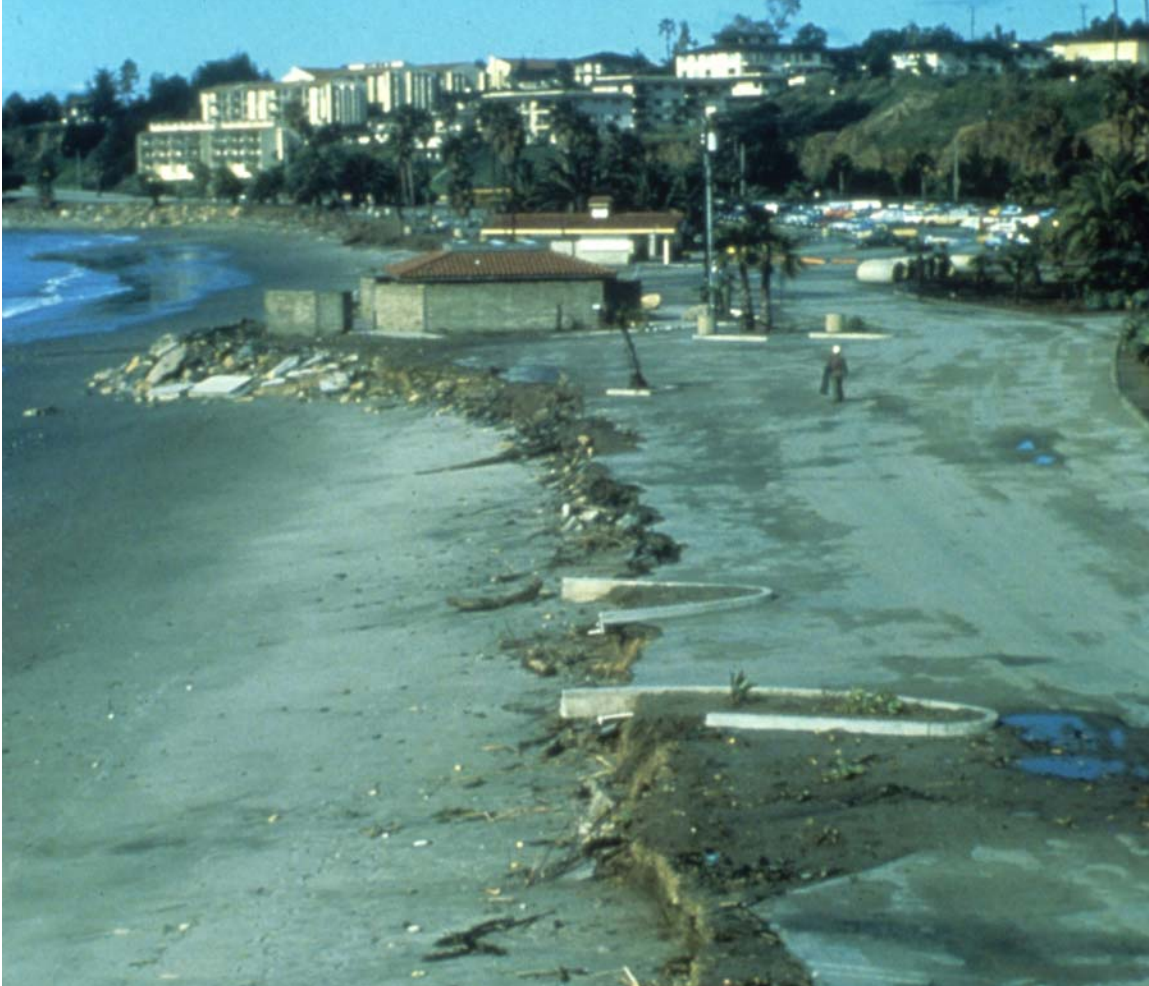
Figure 2.15: Looking West at Erosion That Removed Part of the Leadbetter Beach Parking Lot during the 1983 El Niño
