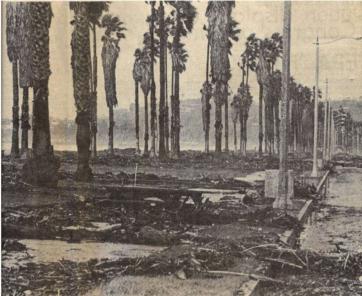
Figure 2.17: Palm Park, along Cabrillo Boulevard, Is Strewn with Debris, Including a Picnic Table That Was Carried in by Waves That Overtopped East Beach in March 1983.
