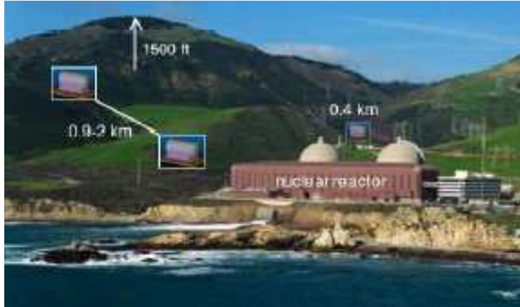
Figure 45: Picture of the Diablo Canyon nuclear power plant in San Luis Obispo County, California, USA. The local topography at Diablo Canyon allows the construction of an underground tunnel between 0.9-2 km for the placement of two or more neutrino detectors. A longer tunnel up to a distance of 3 km is possible. It may be possible to place an additional near detector at 0.4 km under artificial overburden.
