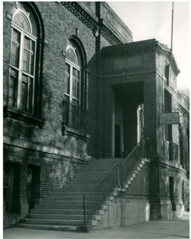
Figure 12: Entrance to Alta Branch Library, Cleveland
