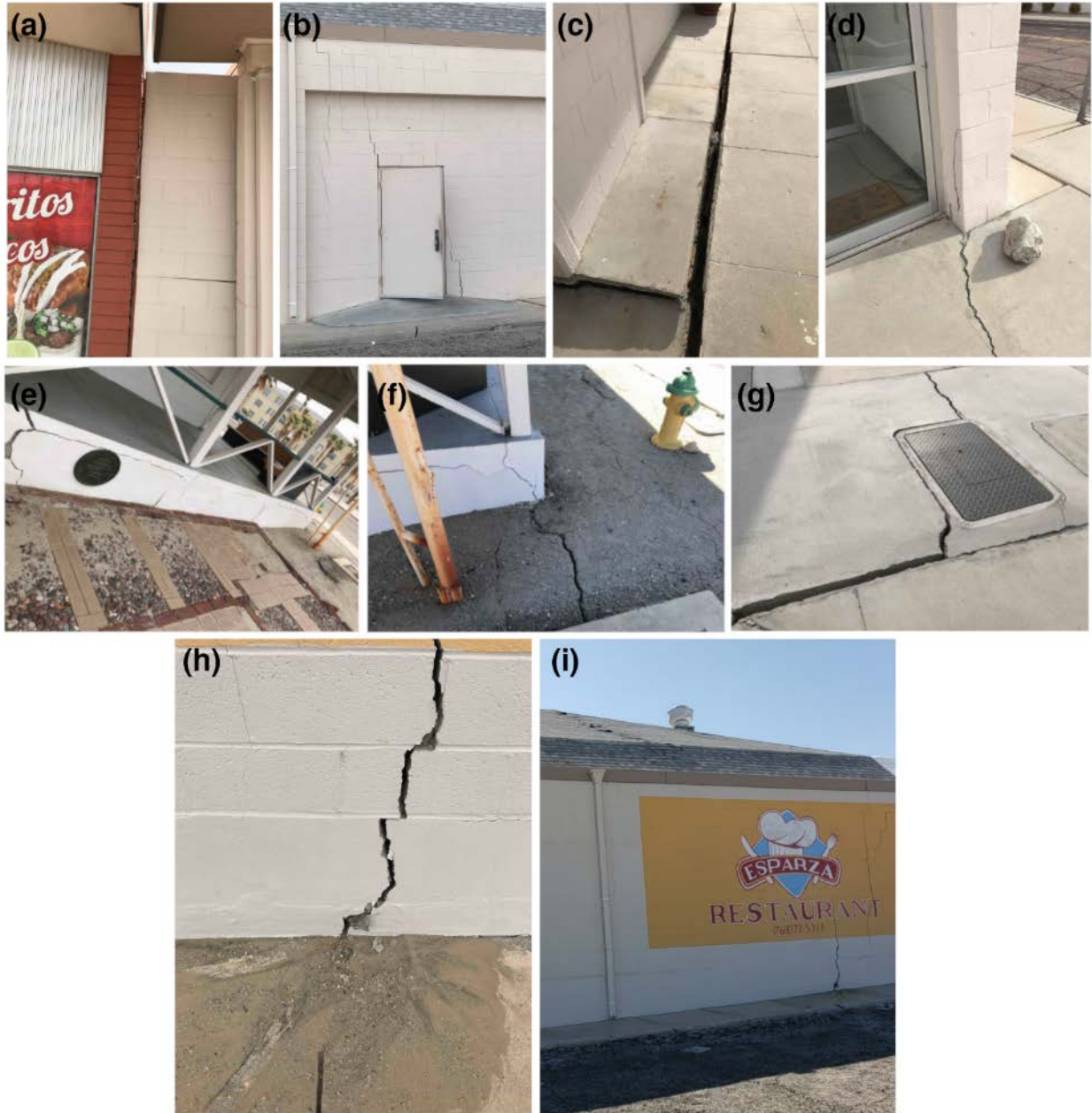
914 Figure 9. Ground failure effects on buildings in Trona. (a) Crack at screen wall between 915 two buildings (35.75979°, -117.376315°). (b, h, i) Wall cracks at the eastern side of the 916 Esparza restaurant with associated sand ejecta and roof damage (35.75957°, - 917 117.37611°). (c, g) Sidewalk pavement crack and offset likely from lateral spreading and
