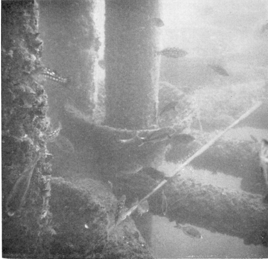
FIGURE 43. Drilling guide cups and cross members at 40-foot depth on "Hazel", showing pipe used as "scratching-post" by fishes. Photograph by Charles H. Turner, March 1960.
