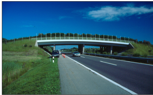
Photo 2. 147.514-km Game Bridge of the M1 Motorway.
