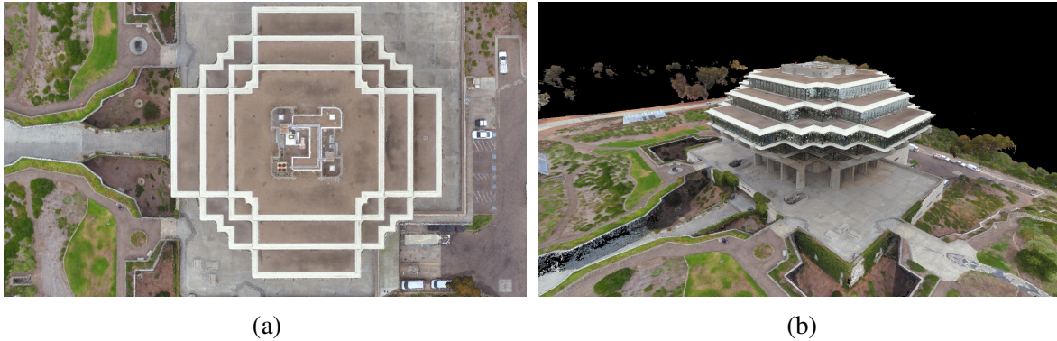
Figure 5.1: Geisel Library baseline UAV imagery, July 28, 2017. (a) View of library rooftop from UAV imagery. North direction is approximately to the right of the image. (b) Additional view of the Geisel Library from baseline UAV survey. The snake head walkway (bottom right of image) is approximately due west of the library structure.
