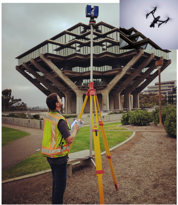
Figure 5.3: Geisel Library LIDAR and UAV survey. LIDAR (main image) survey conducted by KDM Meridian and UAV (inset, top right) survey conducted by the Qualcomm Institute at the UCSD Geisel Library on July 28, 2017.
