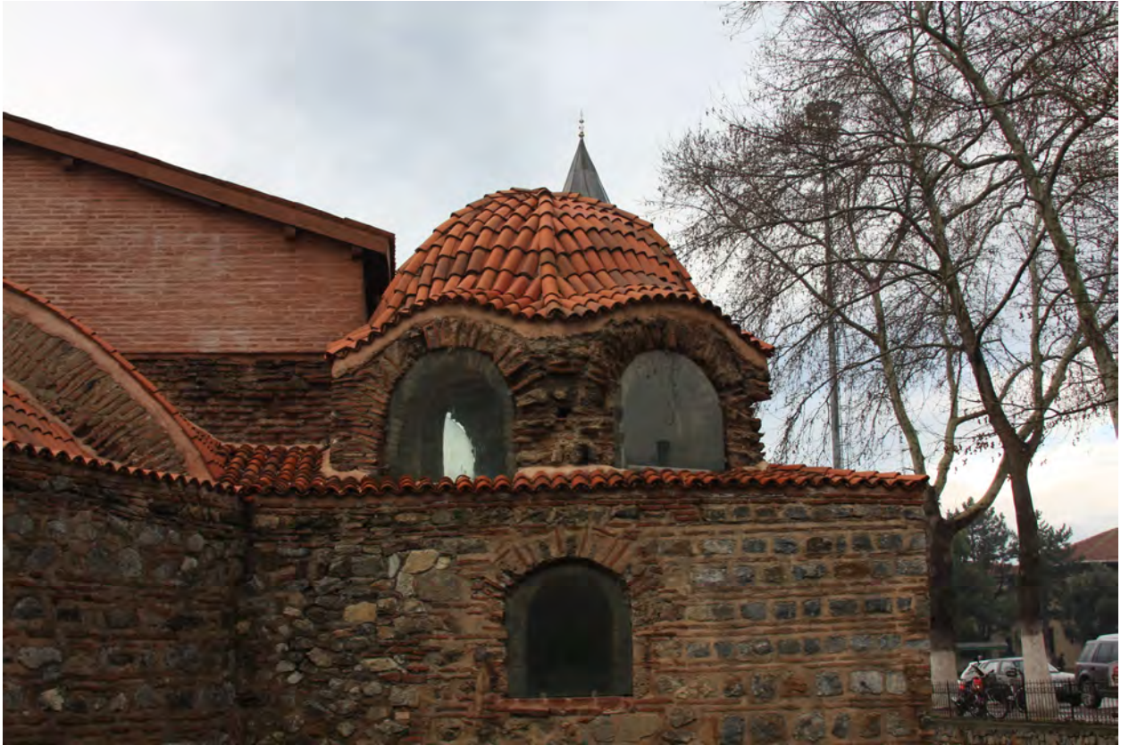
Figure 77: Detail of bonded corners of eastern superstructure, Hagia Sophia, Nicæa (Naomi Pitamber, 2013)
