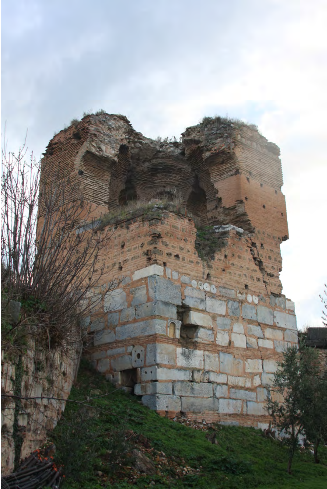
Figure 18: Tower 106, view from inside the city walls (Naomi Pitamber, 2013)
