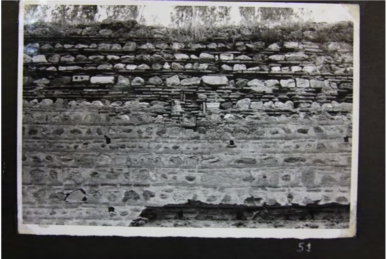
Figure 20: Brick cross immured in Laskarid wall, either between towers 37 and 38, or 38 and 39 (from Bilgiç, "İznik Surları," (The City Walls of İznik), MA Thesis, Art History, İstanbul Univeristy, 1972, Image 51)
