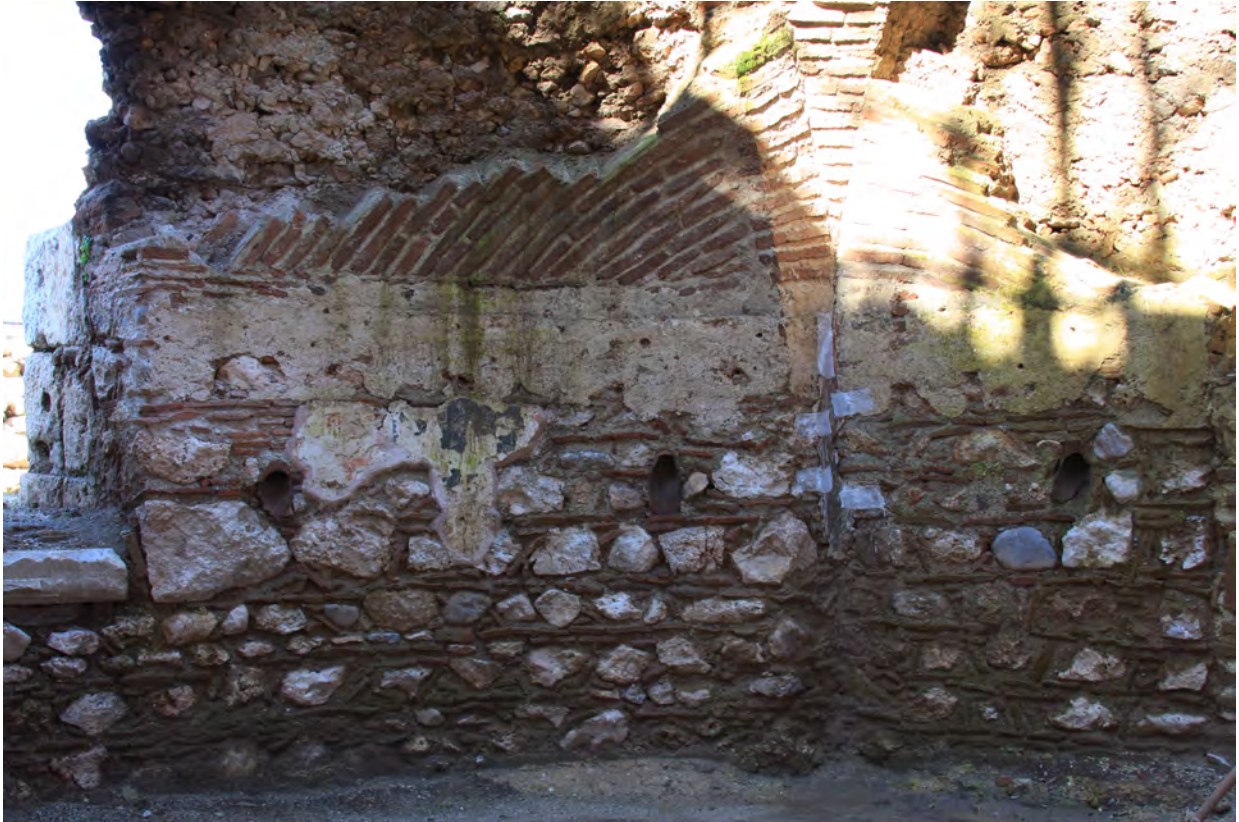
Figure 178: Detail of pipes exiting wall surface, west side, central room, ground floor, Laskarid Palace, Nymphaion (YD Architects, 2013)
