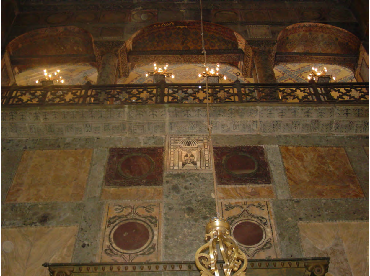
Figure 143: Detail of Marble Revetment decoration immediately above the Imperial Doorway at Hagia Sophia, Constantinople (Naomi Pitamber, 2009)
