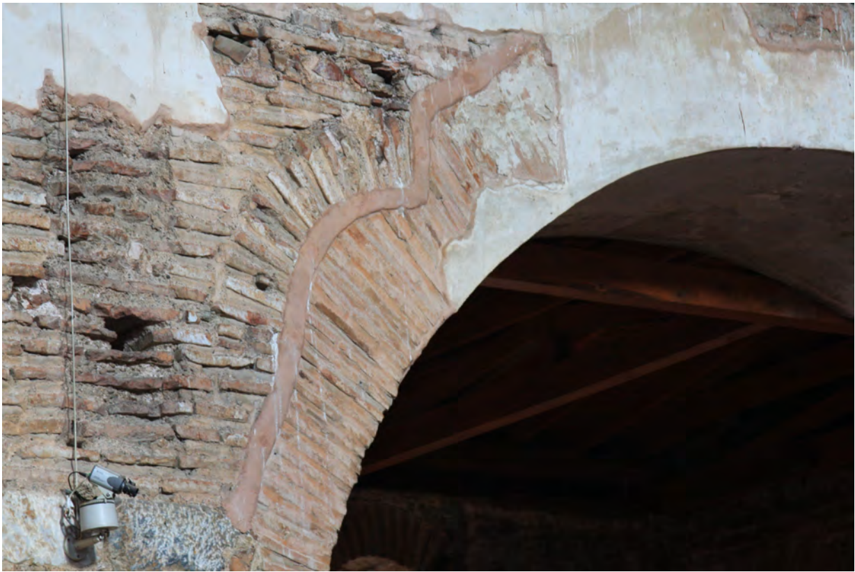
Figure 40: Triple arcade embedded in great arch of Hagia Sophia, Nicæa (Naomi Pitamber, 2013)
