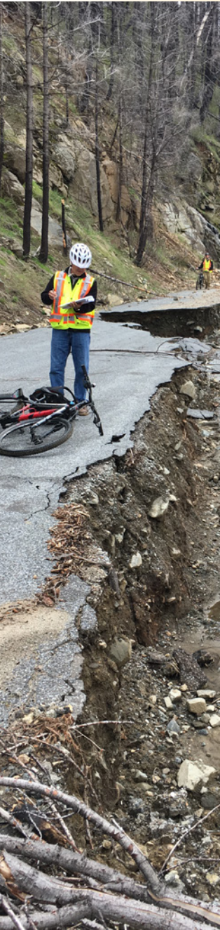
Road damage from postfire soil erosion that occurred in a severely burned area after heavy winter rains. Photo: Vincent Pacific.
