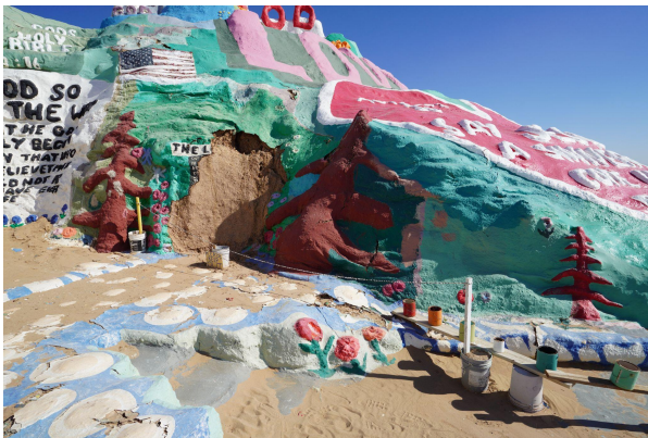
Prior damage to the northern nook, unrelated to the August 2023 storm.
