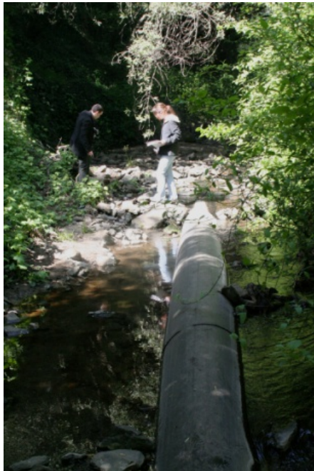
Figure 8. Pressures Photos (sewer lines within the creek, bank erosion, and drop structures blocking fish passage)
