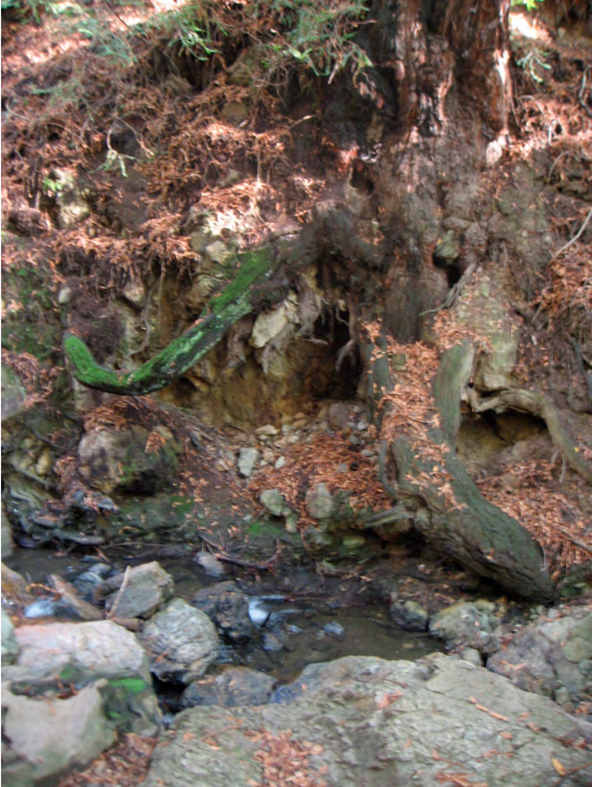
Figure 14: Tree Roots Exposed and bank failure
