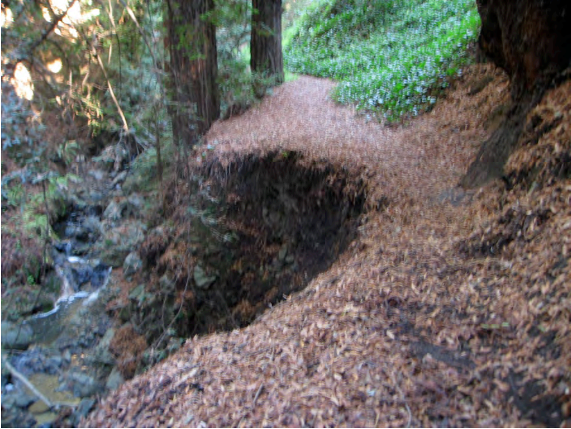
Figure 16: Bank Erosion and Trail Failure
