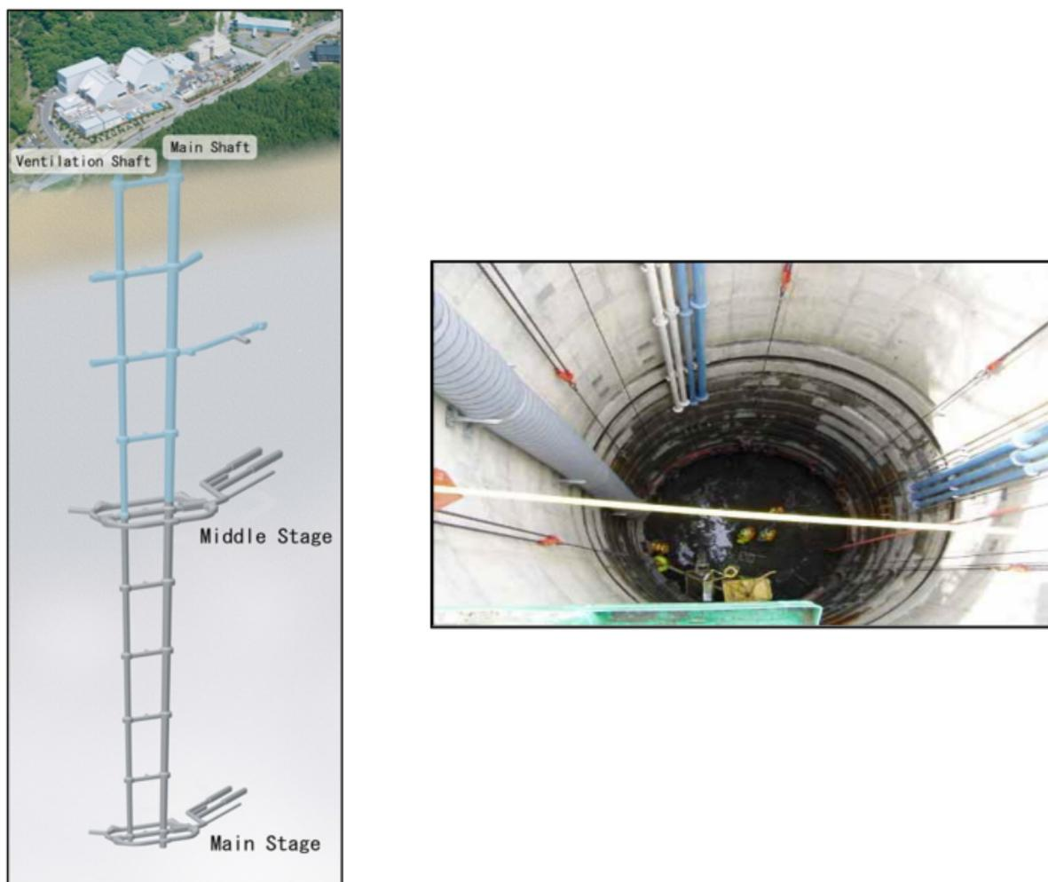
Figure 4.7-1. Layout of the Mizunami Underground Research Laboratory in Japan (left), and photo of tunnel shaft construction (right).
