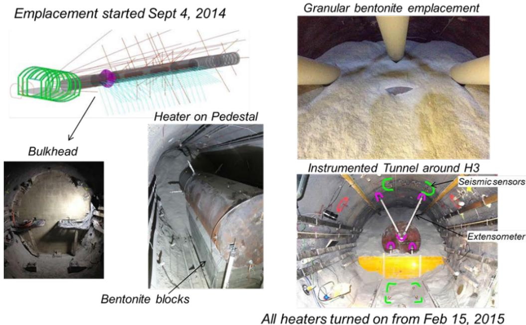
Figure 3.1-8. Images from the construction and installation of heaters, bentonite backfill and plugs (Zheng et al., 2016).
