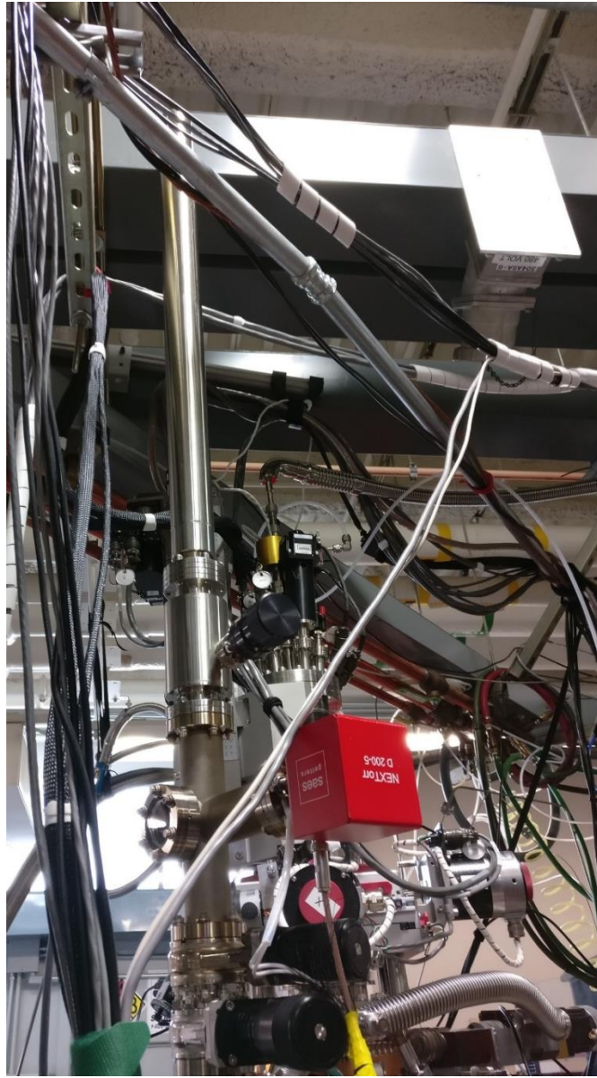
Figure C.2: The ALS vacuum suitcase when installed on the 10.0.1.2 beamline preparation chamber
